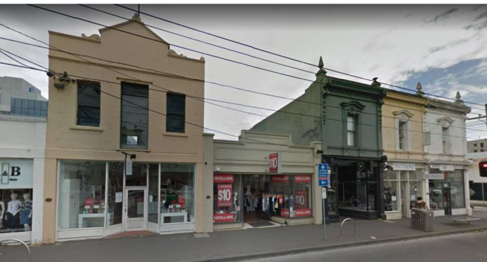
Figure 11. 129-141 Bridge Road, Richmond (Bridge Road Precinct, HO310) (Google, Nov 2016).
