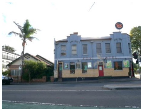
Figure 17: (left) Fox Hotel, 351 Wellington Street and terraced houses, 47 & 49 Alexandra Parade, Clifton Hill ('Contributory' within HO321).
