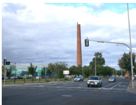
Figure 15: Gasometer Hotel, 484 Smith Street, Collingwood (recommended for inclusion on the Heritage Overlay as an individual heritage place)
