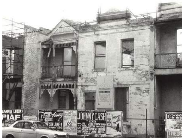
Figure 13. Houses in poor condition on Gertrude Street, 1983 (COYL, Id. FL180).
