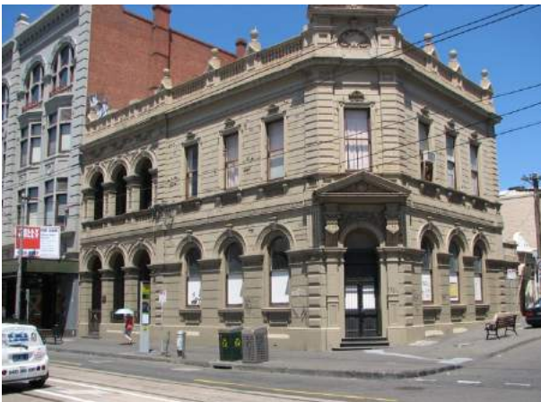
Figure 33. Former Union Bank of Australia, 165-167 Smith Street (VHR H0506) is an example of a local landmark due to its former use as a bank, its prominent corner location and elaborate architectural detailing (VHD, 2008)
