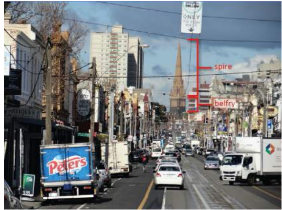
Figure 12. View to St Patricks Cathedral looking south along Brunswick Street.
