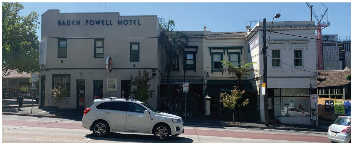
The Baden Powell Hotel (local landmark) and adjoining fine-grain terraces fronting Victoria Parade
