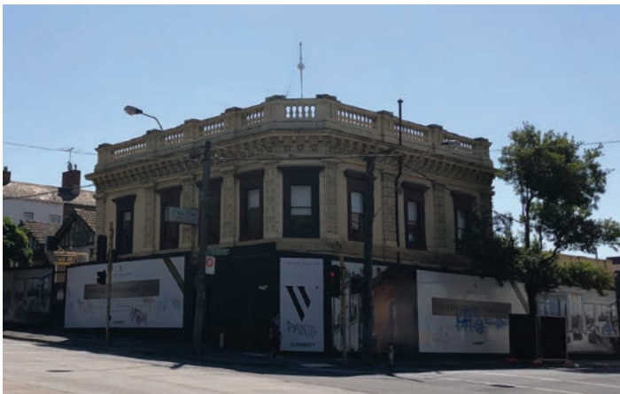
former John Franklin Hotel
