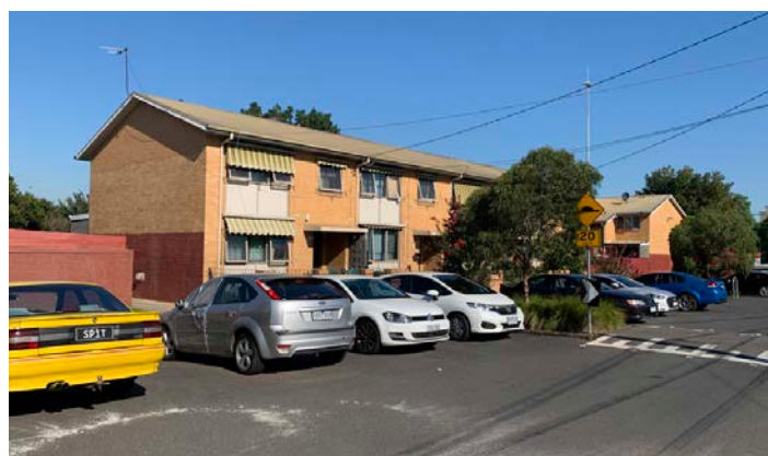
Office of Housing building viewed along Alexander Street
