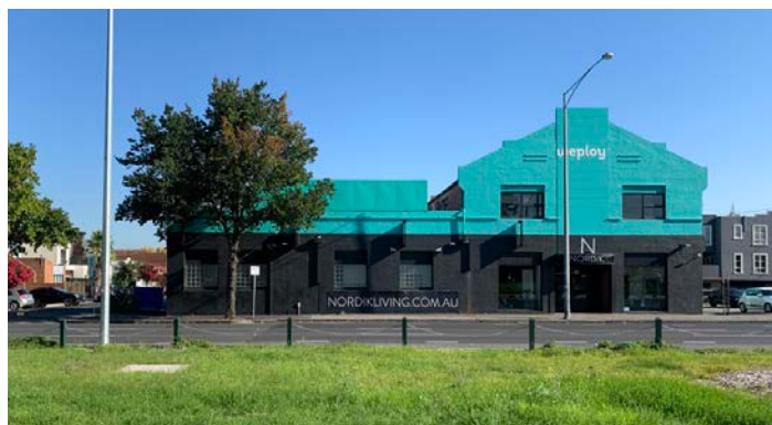
A non-contributory building between Wellington Street and Charlotte Street
