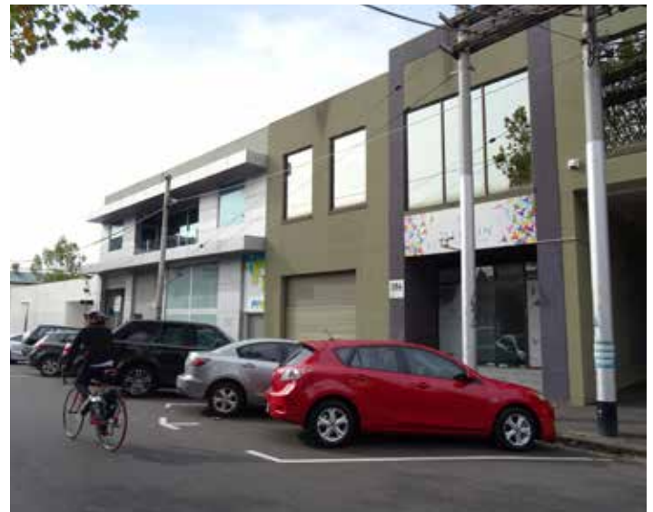
2 storey commercial forms on George Street
