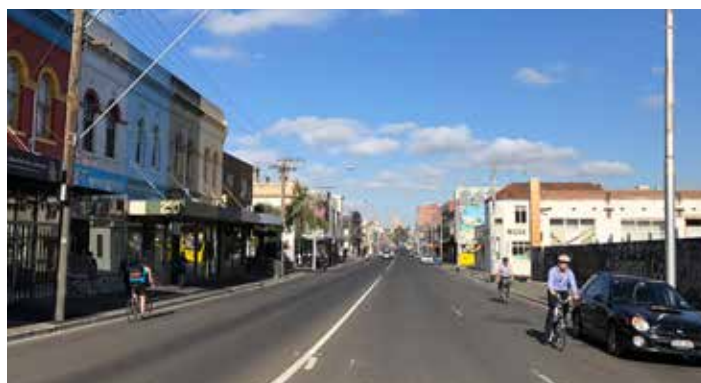
View along Johnston Street towards Redmond Barry building
