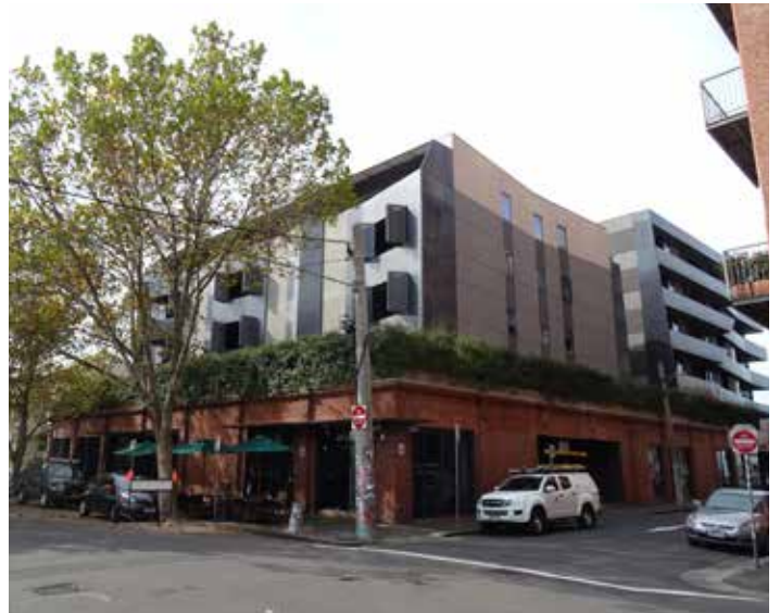
Recent development behind retained heritage facade, Gore and Rose Streets
