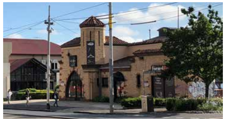
Former Avon Butter Factory at corner of Nicholson Street and Victoria Street
