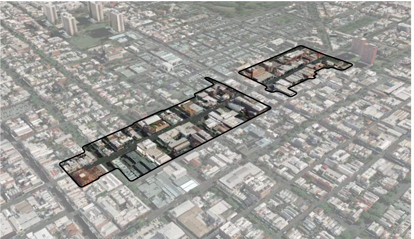
Oblique aerial of Johnston Street Precinct and surrounding context
