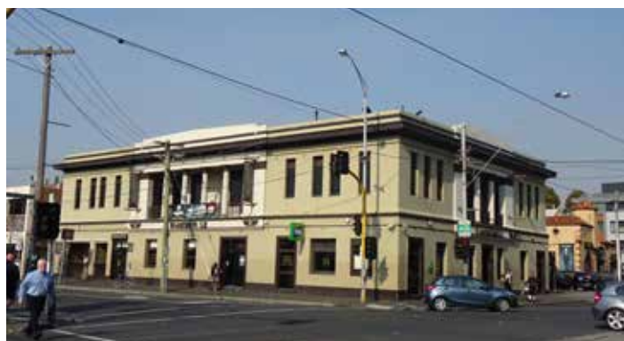
Tankerville Hotel at corner of Nicholson Street and Johnston Street
