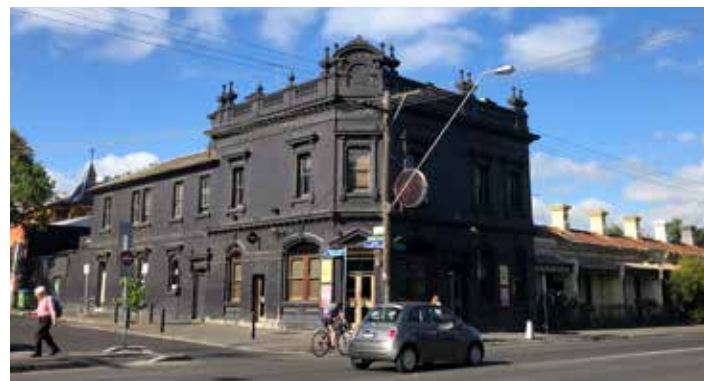
Rochester Hotel at corner Johnston Street and George Street
