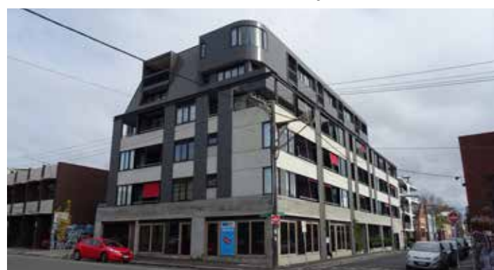
Recent development at corner of George Street and Argyle Street
