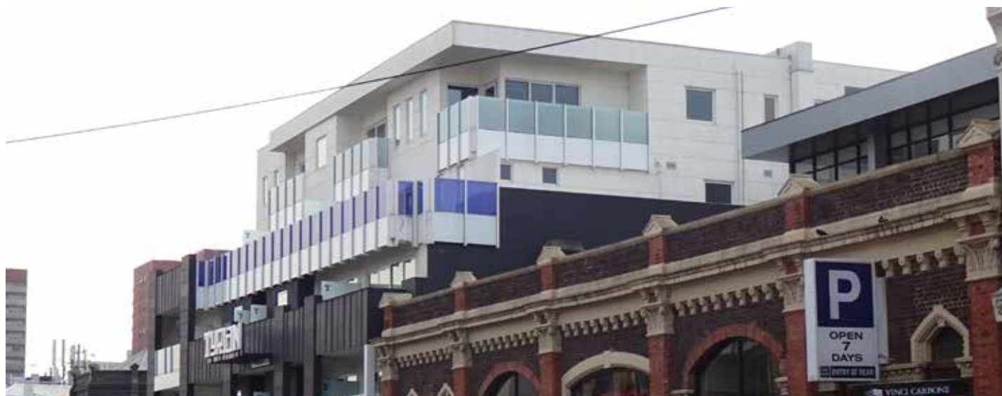
Visually distinct upper levels along northern side of Johnston Street, near Fitzroy Street
