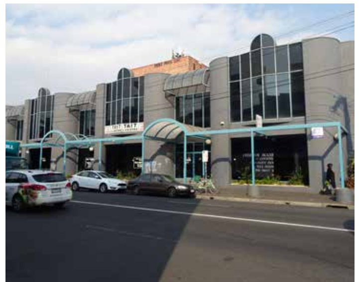
Non-heritage office building 'ripe' for redevelopment
