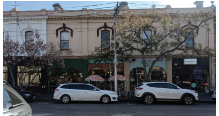
Orderly streetscape between Brunswick and Fitzroy Streets
