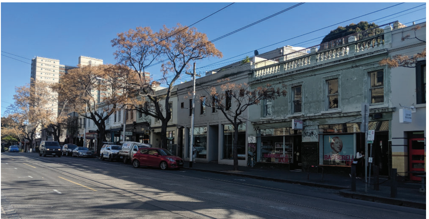
Consistent heritage profile along north side of Gertrude Street
