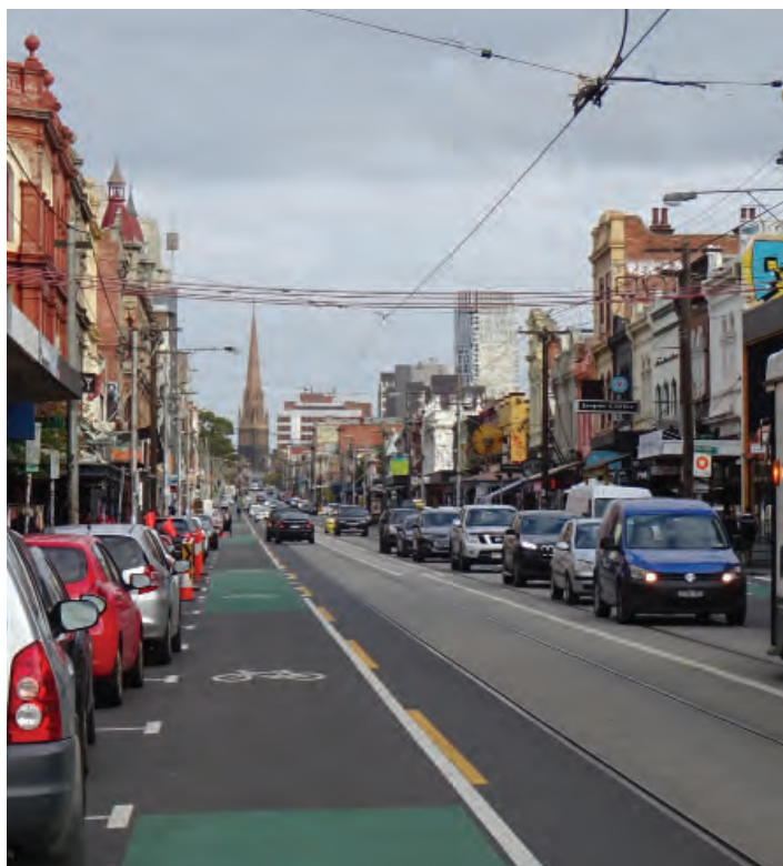
View toward south along Brunswick Street
