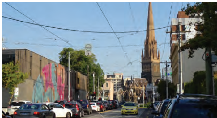
View along Brunswick Street towards St Patrick's Cathedral (looking south)
