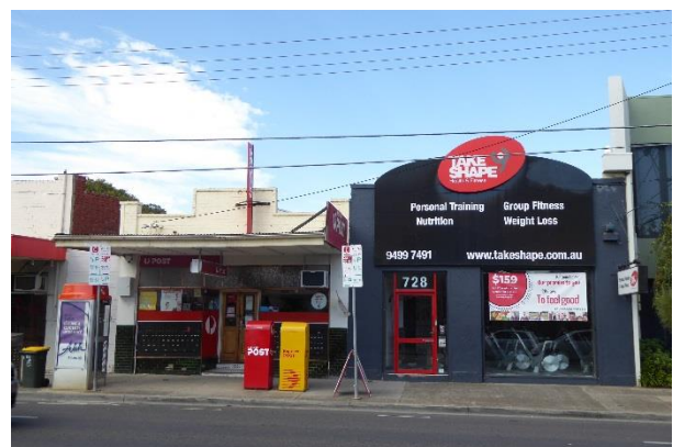
Heidelberg Road elevation – no. 730 (left) and no. 728 (right)
