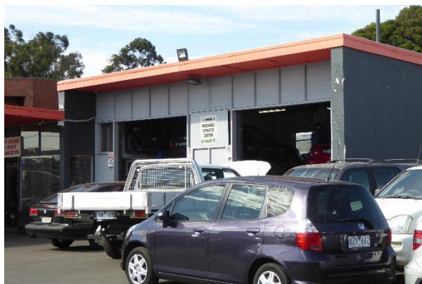
Heidelberg Road - west wing
