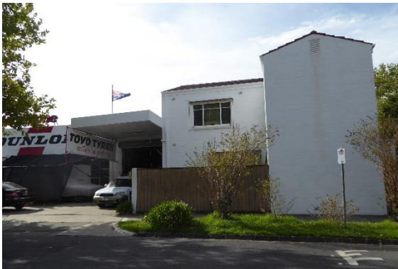
Panther Place (west elevation) – building form and original openings
