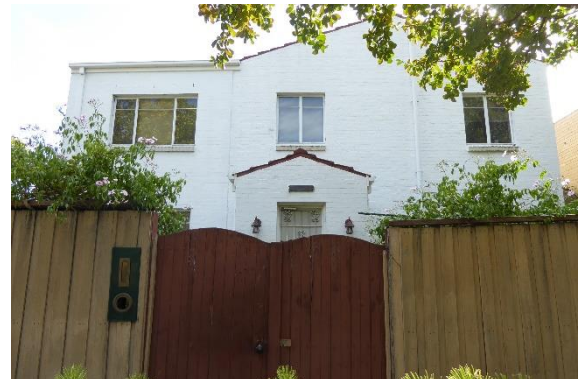
Park Crescent (south elevation) – original openings
