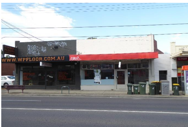
Heidelberg Road elevation – no. 734 (left) and no. 732 (right)
