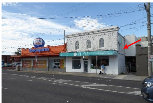
The entire west (side) elevation of the former Butcher Shop (HO71) remains exposed
