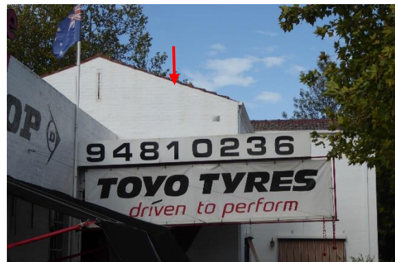
Heidelberg Road – original roof form of house is visible
