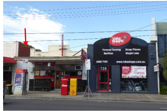
No. 732 – the original parapet and west return are visible from Heidelberg Road
