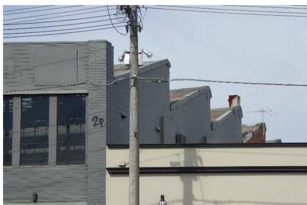
Sawtooth roof forms from Heidelberg Road
