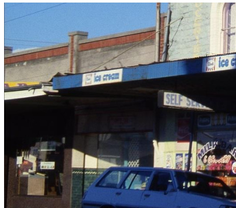
1982 image – showing original parapet detailing
