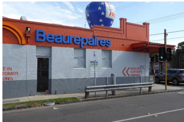
Yarralea Street (east) elevation
