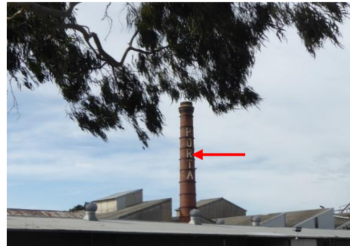
Retain view/sightline of integrated 'PORTA' sign on chimney from the street
