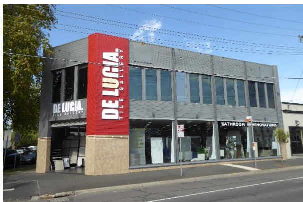
Heidelberg Road (north) elevation
