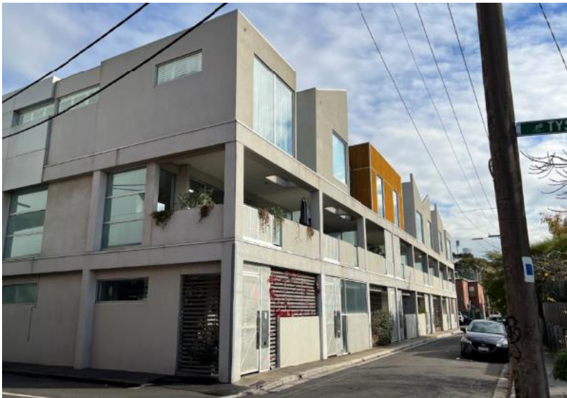
Figure 18: View south-west to No. 4-16 Tanner St Margaret St (Source: Officer photo May 2022)
