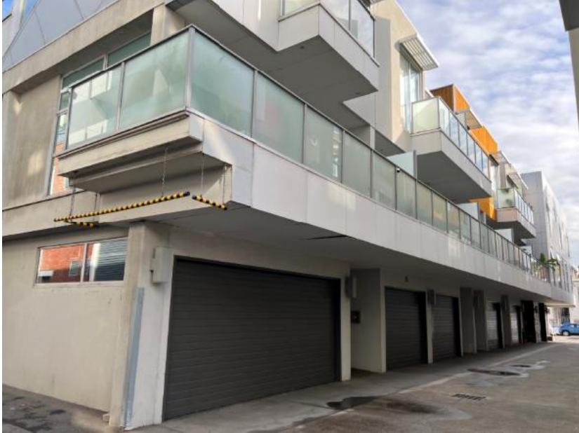
Figure 17: No. 4 Margaret St northern elevation and private driveway (Source: Officer photo May 2022)
