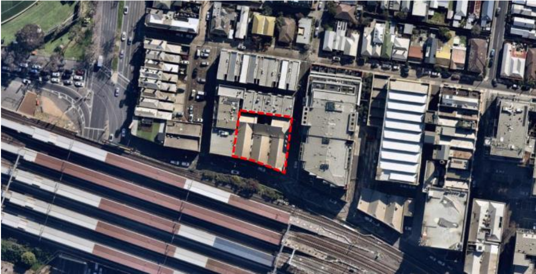
Figure 11: Aerial Photo of subject site and surrounds (Source: Contour Town Planning Report)
