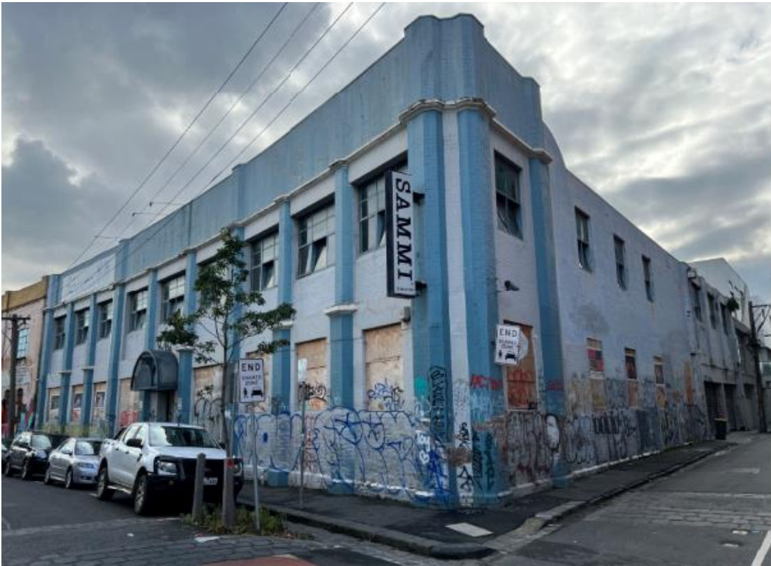
Figure 12: Photo of subject site showing the Stewart St and Margaret St frontages (Source: Officer photo May 2022)
