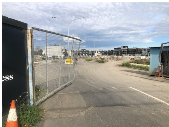
Figure 12: Existing entrance to Mills Boulevard from Heidelberg Road.
