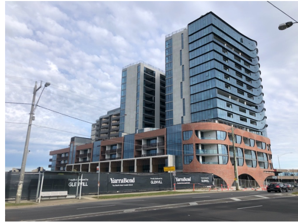
Figure 14: Existing built form west of the review site, at the Heidelberg Road frontage.
