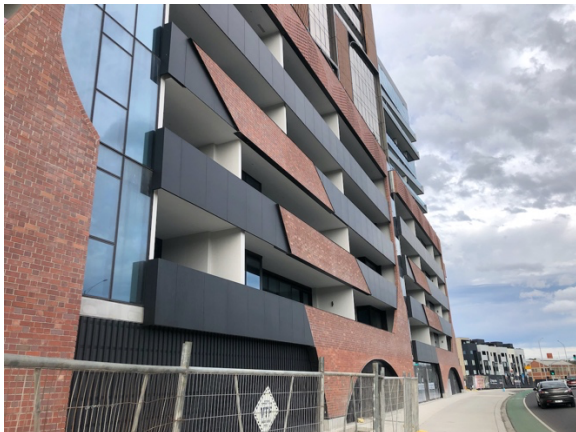
Figure 05: Chandler Highway podium frontage.
