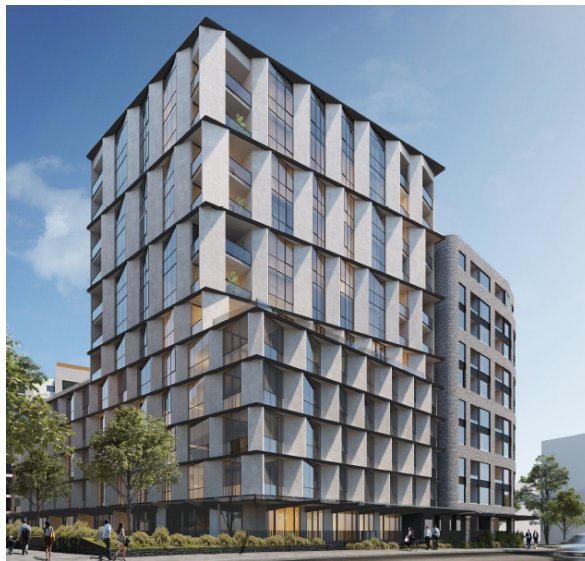
Figure 7: North-west corner view from Chandler Hwy (Building A and B)
