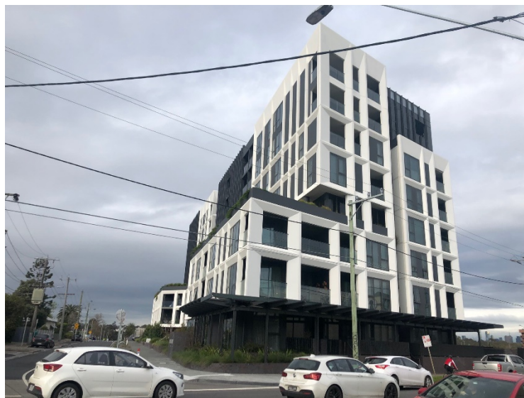
Figure 2 – 680 Heidelberg Road PLN17/0272 as constructed
