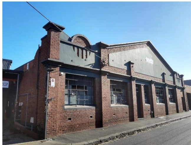
Figure 5: Subject site – Northern portion – former Davis' Pickle and Sauce Factory
