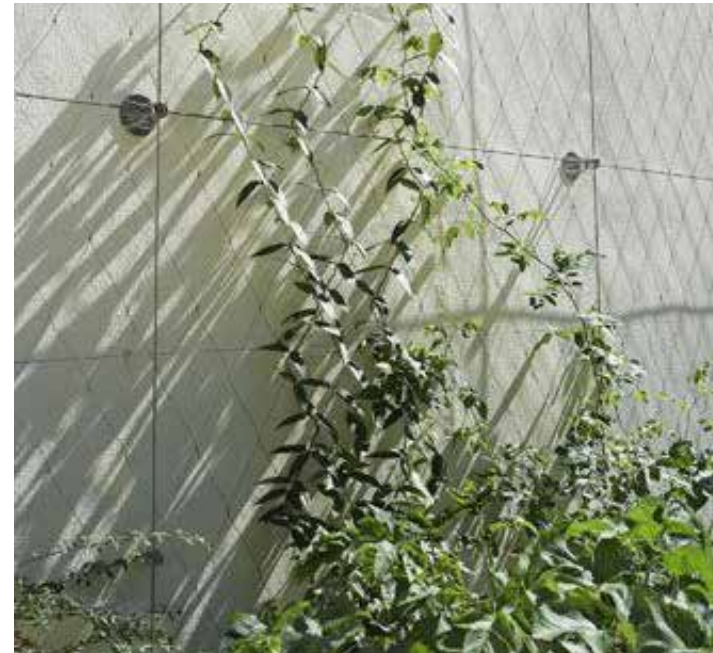
EN-03 Tensile wire for planting
