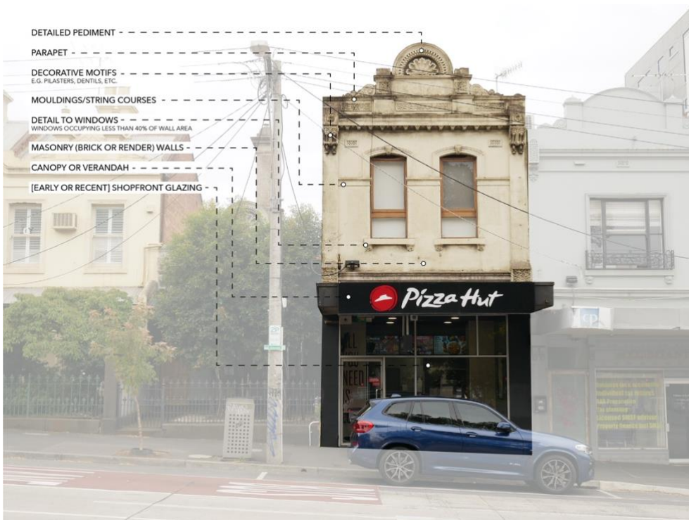
Figure 35: Shop / Residence (27 Victoria Parade, Collingwood, within HO336)
