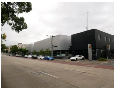
Figure 28: (left) Houses, 71-73 Victoria Parade ('Contributory' within HO336); former John Franklin Hotel, 75-77 Victoria Parade, Collingwood ('Individually significant' within HO336)
