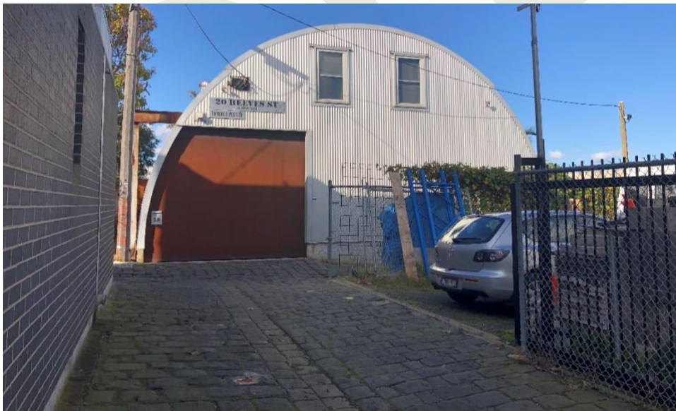
Figure 13. West elevation of the structure, showing later window suites above the sliding door.
