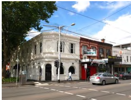
Figure 32. (left) Shop, 295 Victoria Street, Abbotsford (HO56)
