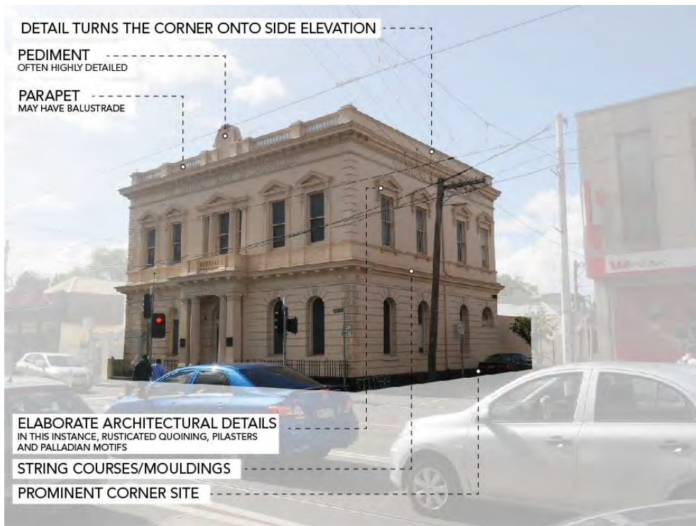
Figure 33. Major commercial building typology, showing typical features. This example is the Former National Bank, located within Precinct 3 at the northwest corner of Victoria Street and James Street (address 261 Victoria Street, Abbotsford). Other examples of prominent commercial buildings may include pubs or hotels.
