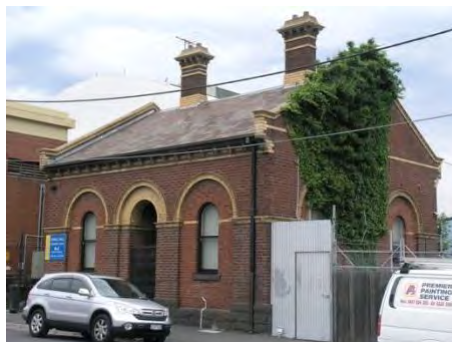
Figure 57. (left) North side of Bridge Road looking west from the intersection with Gardner / Lord streets, 433 Bridge Road on the right (part HO310)
