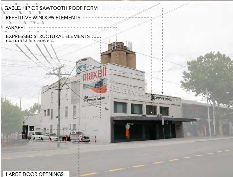
Figure 13. Industrial building typology, showing typical features. This example is the Former Flour Mill & Grain Store, located within Precinct 4 on the southern side of Bridge Road at 534 Bridge Road.
