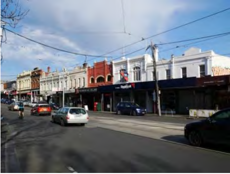
Figure 20. (left) Looking west down the southern side of Bridge Road from Hoddle Street (HO310)
