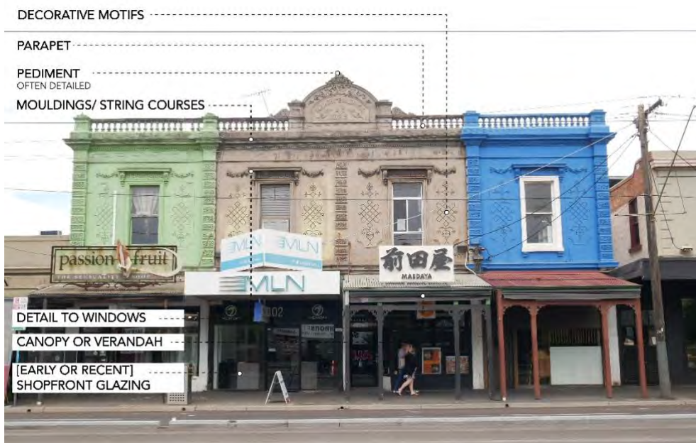
Figure 10: Shop/residence typology diagram, showing key features. Some variation between examples is typical. This example is located within Precinct 2 (address 398 – 404 Bridge Road).
