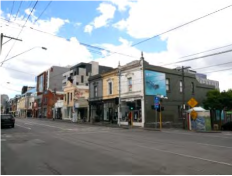
Figure 22. (left) South side of Bridge Road (112 Bridge Road on the right) (HO310)
