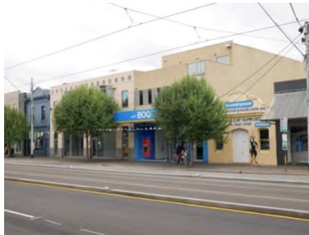
Figure 55. (left) North side of Bridge Road looking east from the southeast corner of the intersection with Coppin Street, 403 Bridge Road on the left (HO310)
