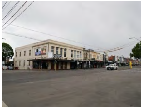
Figure 37. (left) South side of Bridge Road looking east toward Coppin Street, 350 Bridge Road on the right (HO310)
