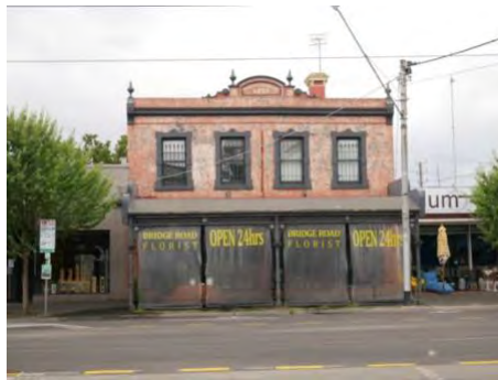
Figure 81. (left) Northeast corner of the intersection of Bridge Road and Burnley Street, Royal Oak Hotel, 527 Bridge Road (HO529 and HO310)
