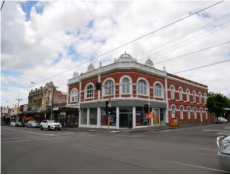
Figure 24. (left) South side of Bridge Road looking west from the intersection with Lennox Street (170 Bridge Road on the right) (HO310)
