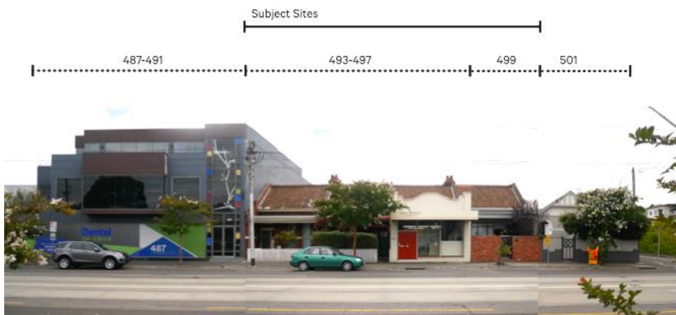
Figure 1. The study area (487-501 Swan Street) viewed from the southern side of Swan Street. The subject sites are numbers 493, 495 and 497 Swan Street. (Source: Hodyl & Co, March 2021).
