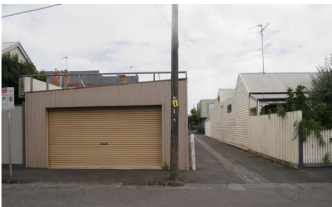
Image 3. View from the west along unnamed laneway to the rear of the Subject Sites. The buildings to the north have side interfaces oriented to the laneway.
