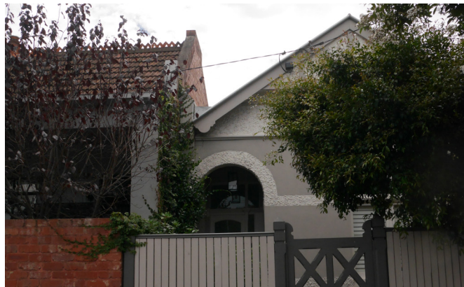
Image 2. Boundary interface between 499 Swan Street and 501 Swan Street - single-storey residential building with a pitched roof form that directly abuts the site. Front setbacks are generally in alignment.
