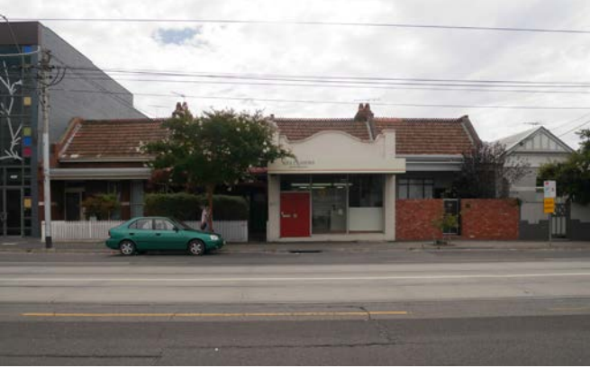
Image 7. View from the south demonstrating ridgeline of the southern roof slope (with decorative tiles) facing Swan Street.
