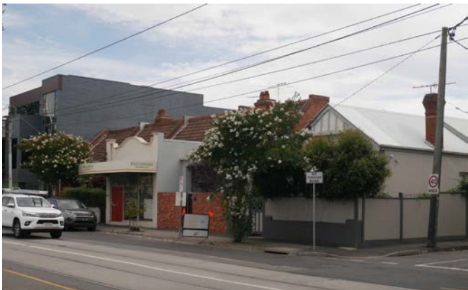
Image 1. View of the Subject Sites from the south-west. Demonstrates varying setbacks from the street, roofline and interfaces with neighbouring buildings to the east and west.
