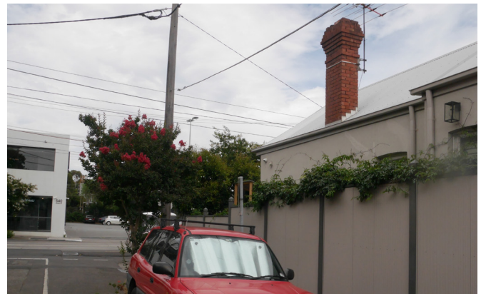
Image 12. View of the chimney at 501 Swan Street from Queen Street.
