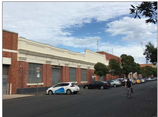
Figure 9. former Foy & Gibson Complex (east side of Cambridge Street) (HO318)
