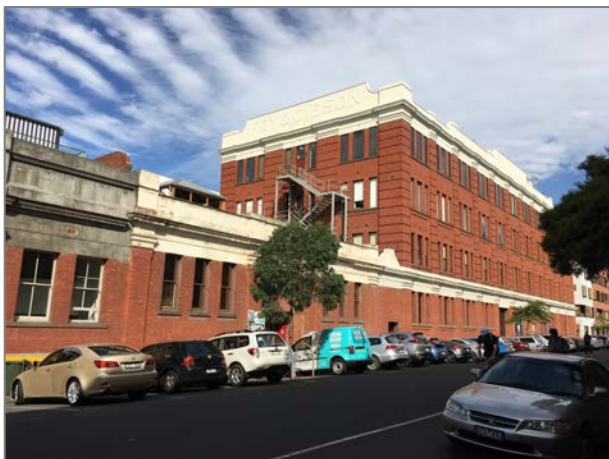
Figure 5. former Foy & Gibson Complex (east side of Oxford Street) (VHR H0755)
