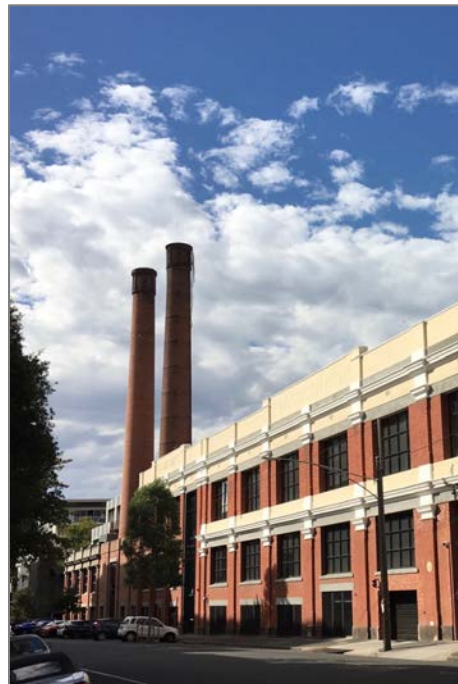
Figure 6. Twin chimneys at the northern end of the former Foy & Gibson Complex (VHR H0755)
