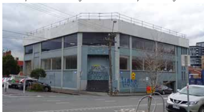
Development site at corner Oxford and Langridge Streets
