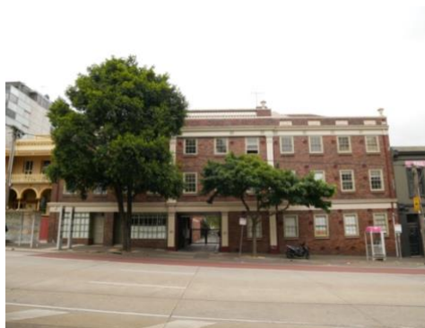
Figure 24: Shop / residences, 27-37 Victoria Parade, Collingwood ('Contributory' within HO336)
