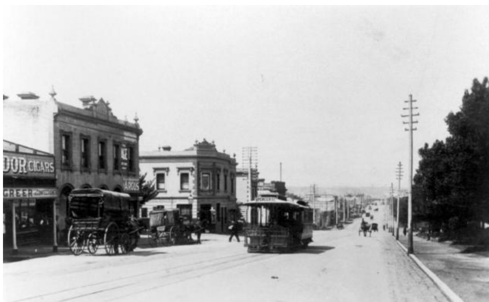
Figure 4: Looking east down Victoria Parade, near the corner of Cambridge Street, Collingwood. Photo dated c1906-c1918 (COYL, Image CL PIC 594)
