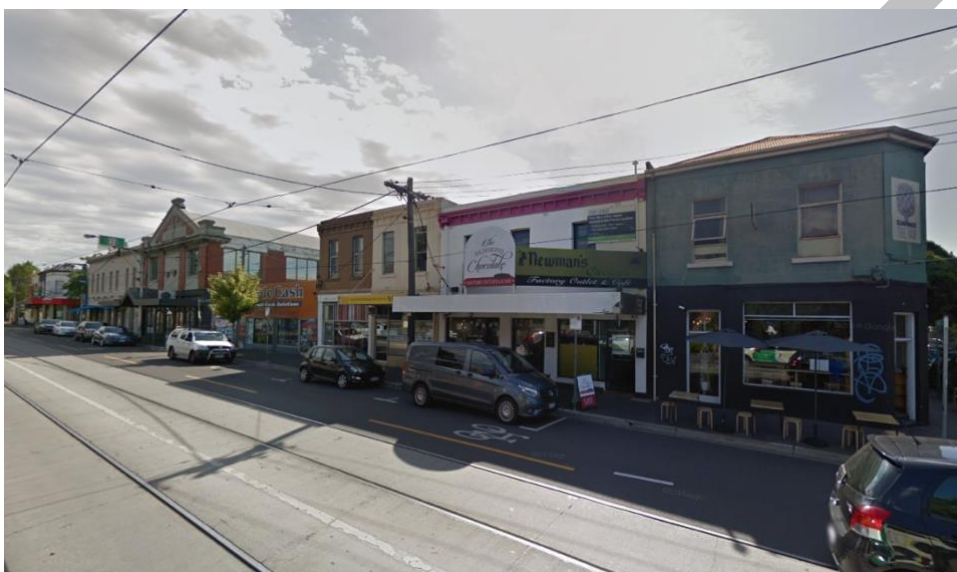
Figure 13. 97-135 Church Street, Richmond (Church Street North Precinct, HO454) (Google, Oct 2016)
