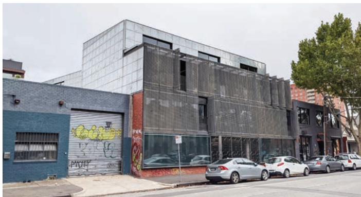
Recent 4 storey development along Kerr Street
