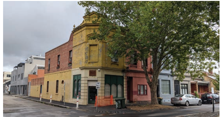
Contributory dwellings along Westgarth and Fitzroy Streets
