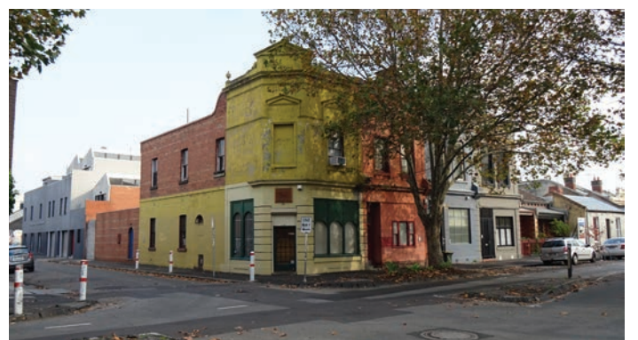
Corner profile of Westgarth and Fitzroy Street
