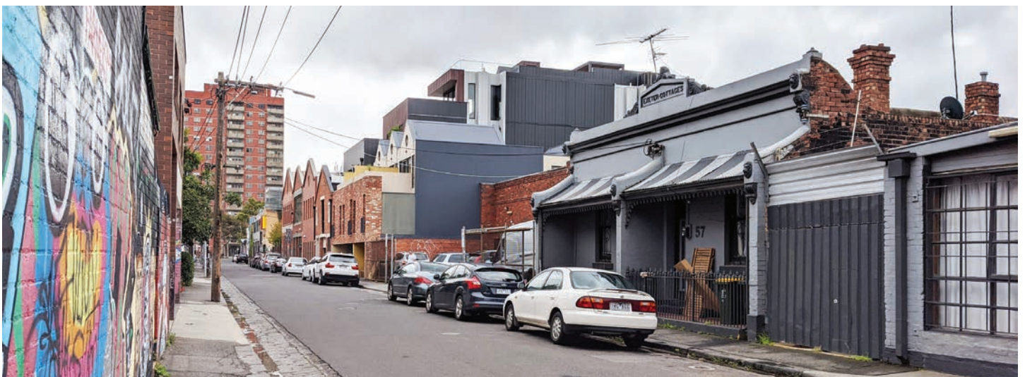
View of varied built form along Argyle Street
