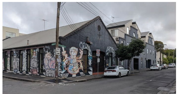
Individually significant warehouse along Leicester Street
