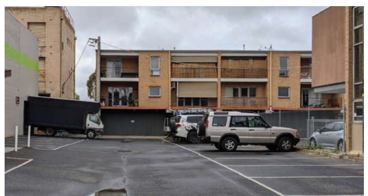
C2Z site on Nicholson Street with interface to NRZ
