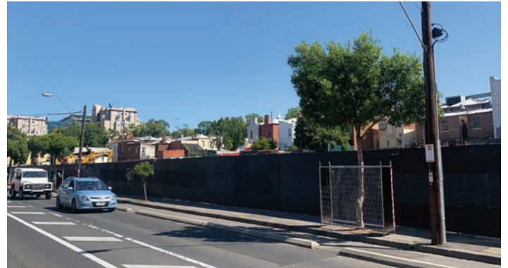
Land undergoing development in the adjoining Collingwood Mixed Use Precinct
