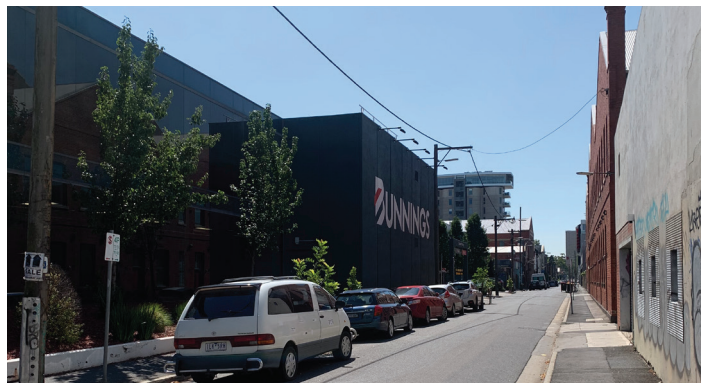
The triple fronted Bunnings allotment as viewed along Islington Street
