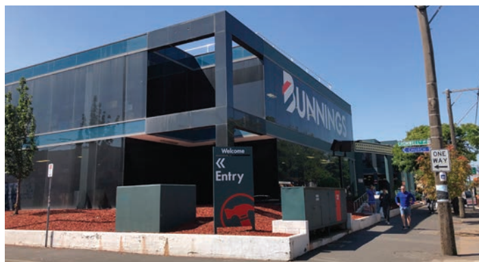
Commercial warehouse extending between Cromwell and Islington Streets
