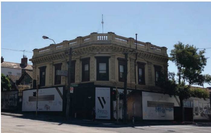
former John Franklin Hotel
