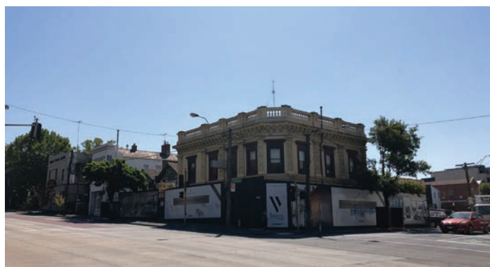
Southwest corner of the Wellington Street junction undergoing change
