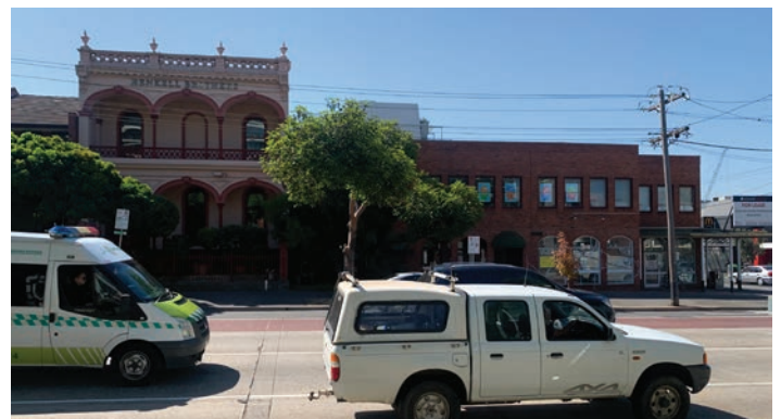
The VHR listed Henkell Brothers terrace adjoining a site with no heritage value
