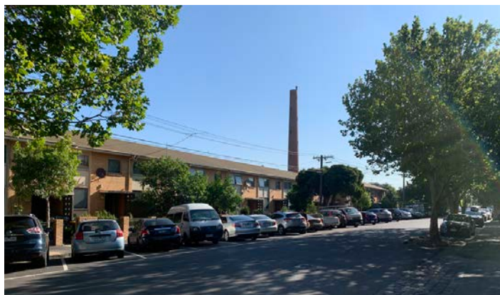
Existing conditions along Noone Street within Precinct 3
