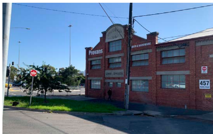
The heritage fabric of the former Murray Co. Wool Works building
