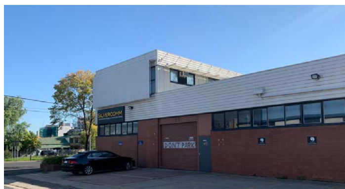
Example of a broad frontage warehouse on the northern side of the Parade
