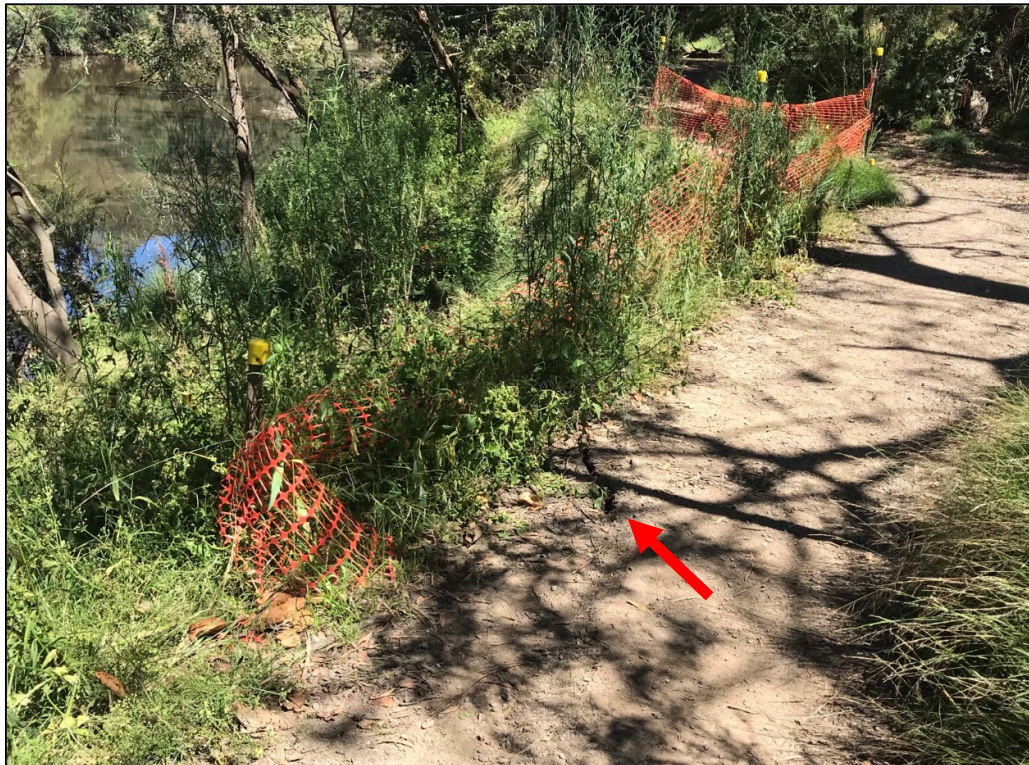
Image 2. Looking west, with arrow pointing to the largest of the newly appeared soil cracking, next to the existing para-webbed exclusion zone.
