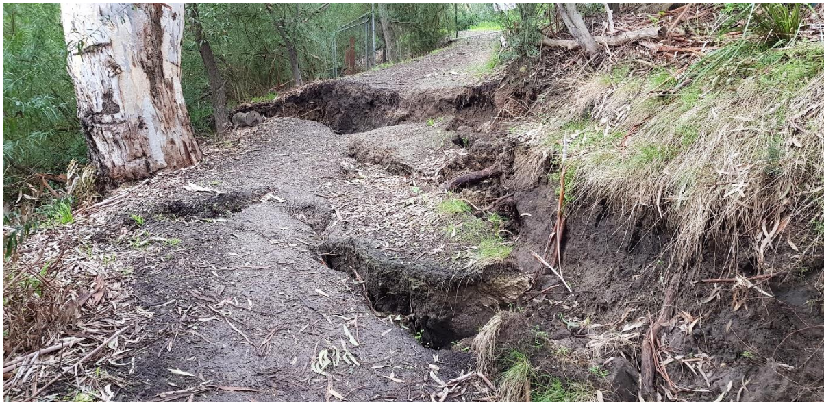
Figure 2. Tree (T1) and bank slump site visit by Alluvium (August 2019)
