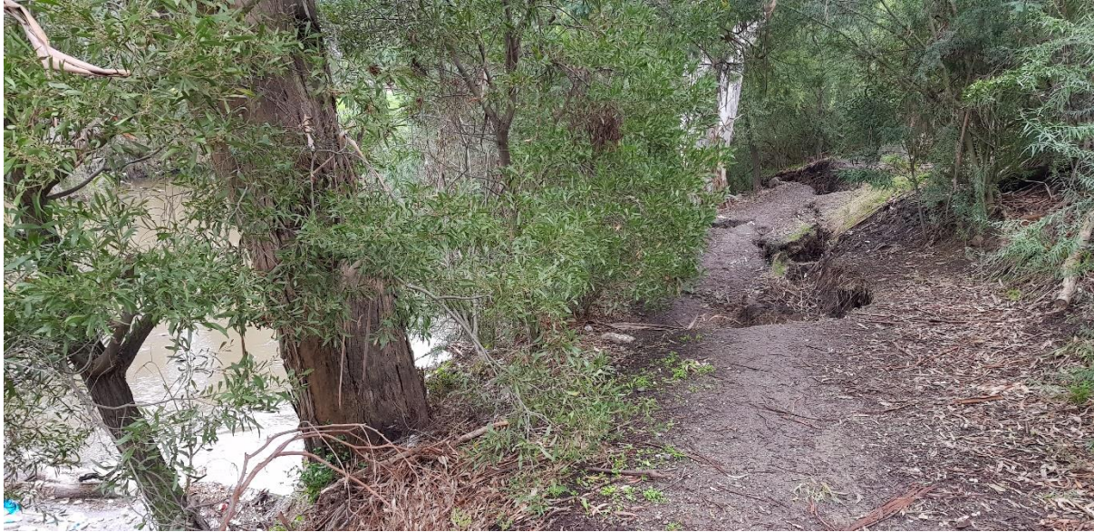
Figure 3 Tree collapse (T2) at the edge of bank slump (August 2019)
