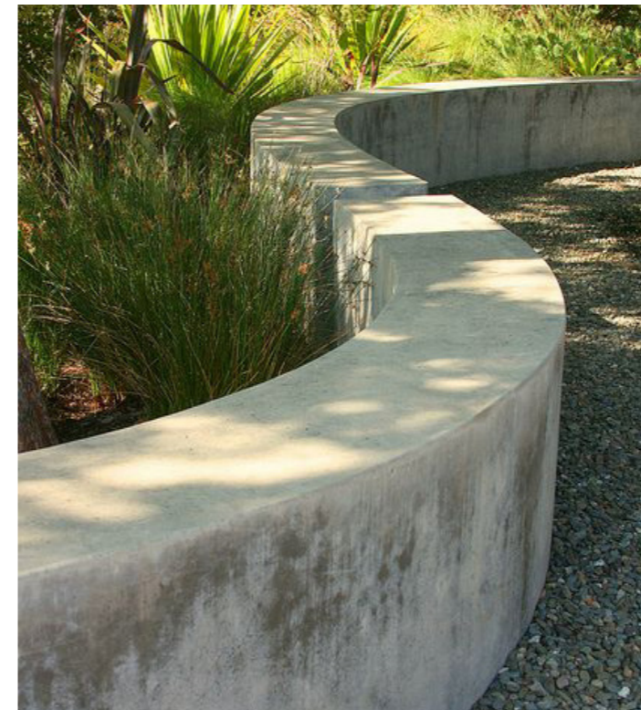
Low concrete wall to gardenbed
