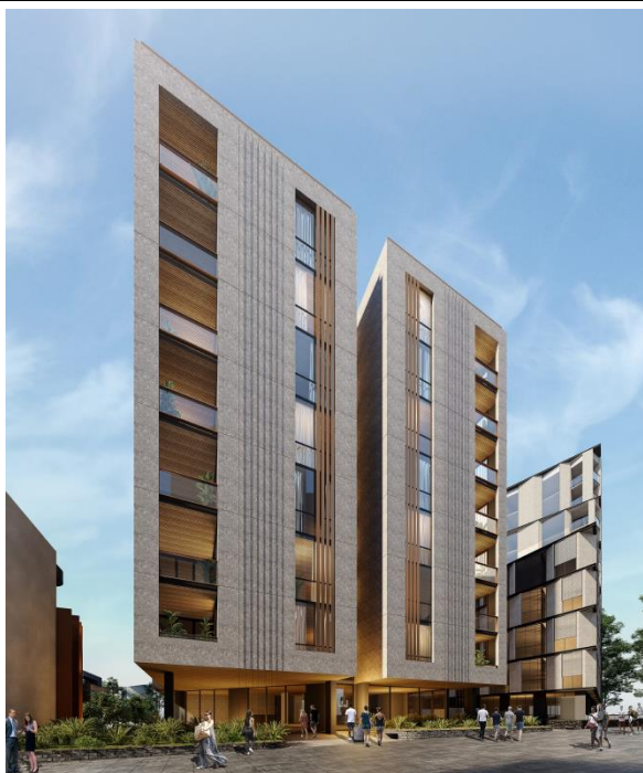
Figure 7 – Northern View of Building D
