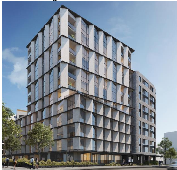
Figure 5 –North-west corner view from Chandler Hwy (Building A and B)
