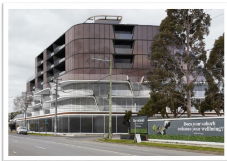
Figure 21: Application PLN17/0040 for 700-718 Heidelberg Road, viewed from the corner of Parkview and Heidelberg Roads
