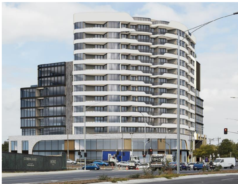
Figure 18 – Application PLN17/0585 for 582 Heidelberg Road, viewed from the corner of Chandler Highway and Heidelberg Roads
