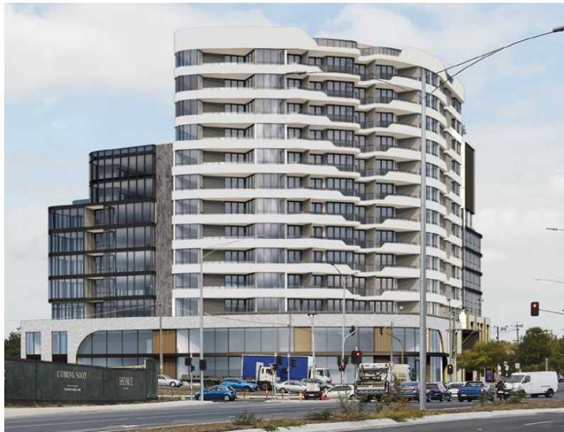
Figure 15 – Application PLN17/0585 for 582 Heidelberg Road, viewed from the corner of Chandler Highway and Heidelberg Roads
