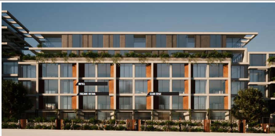
Figure 35 – Building B with variation in treatment between the podium and upper levels
