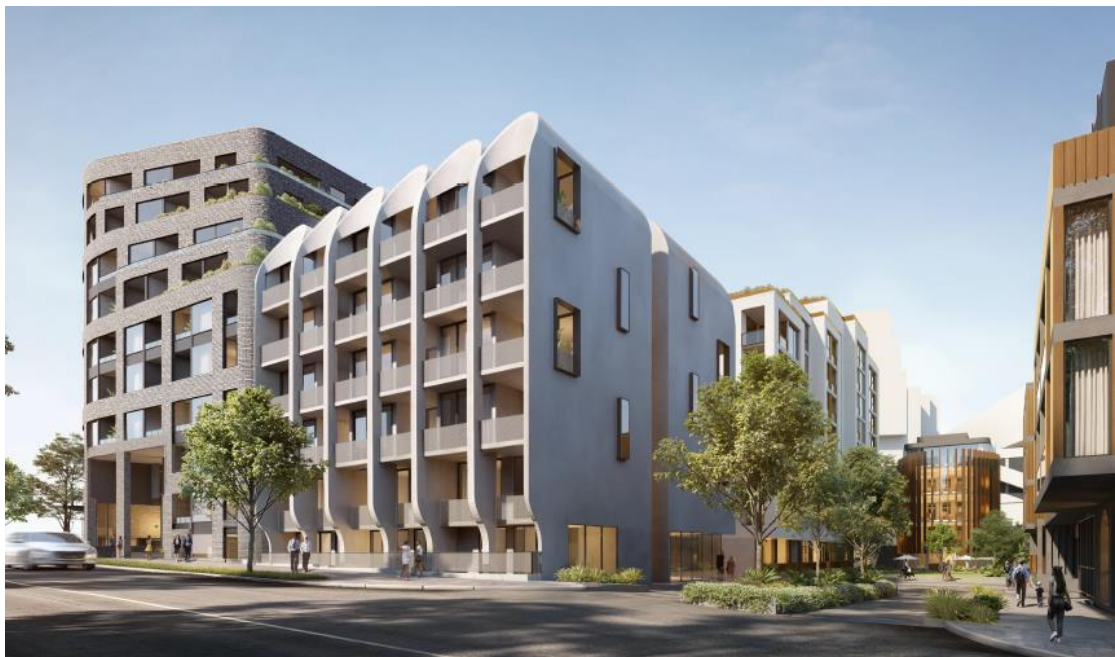
Figure 6 – South-east corner view from Mills Boulevard (Building C, B and D)
