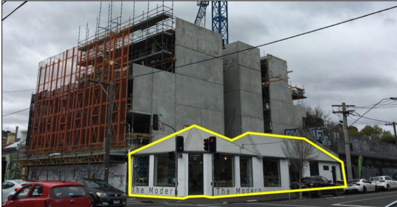
No. 176 Johnston Street Fitzroy (Council Heritage Advisor, August 2020)
