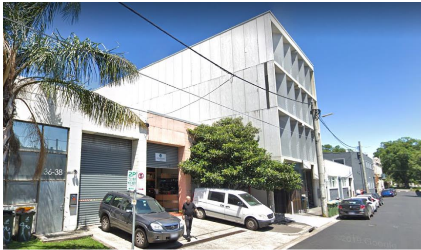
Figure 19: Properties addressed to Rokeby Street to the immediate south.
