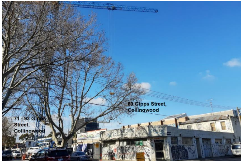
Figure 14: South-east corner of Gipps and Rupert Street, with the land at 71-93 Gipps Street, in the background cleared and cited with a crane in preparation of construction.
