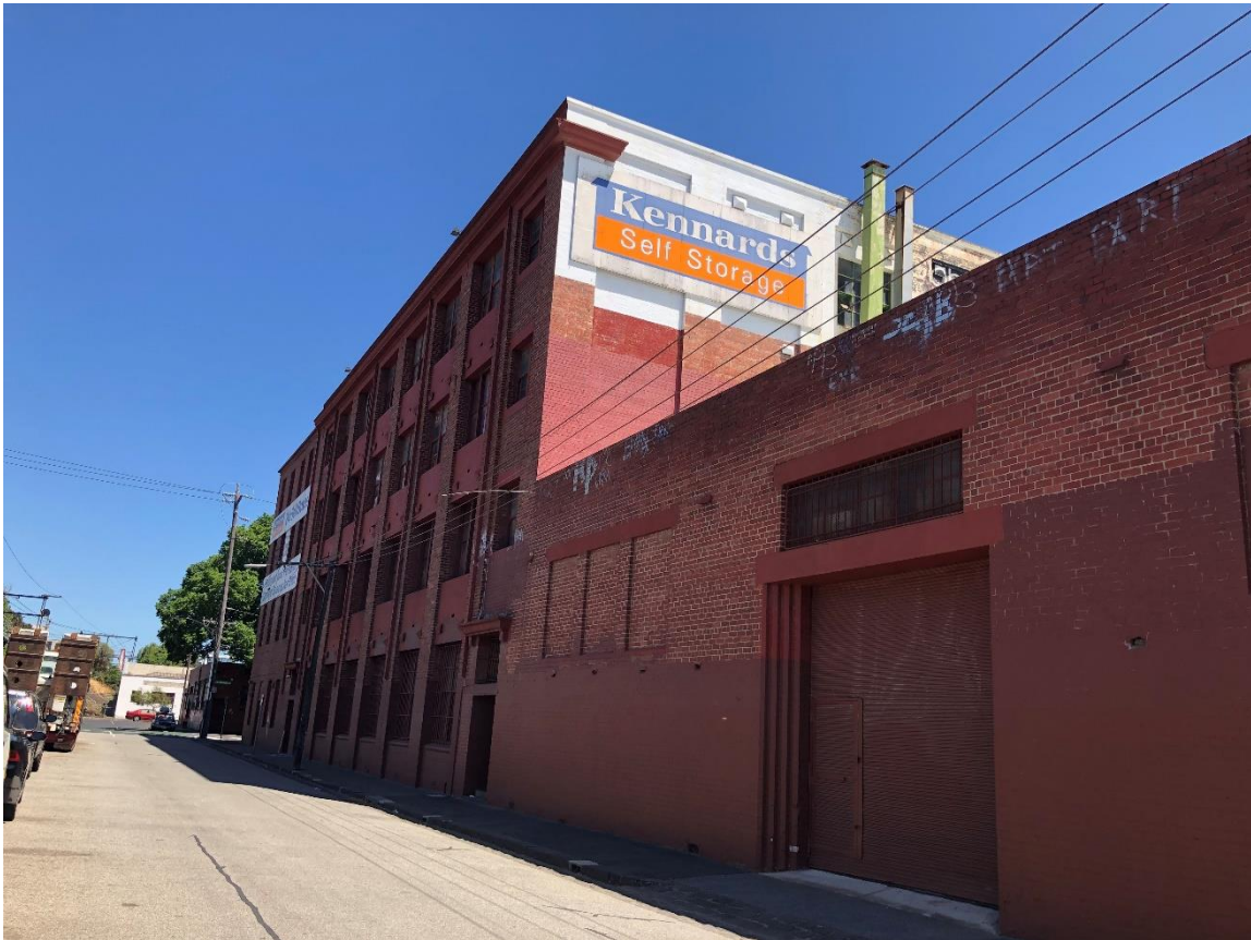
Figure 2: Four storey buildings at 1-15 Russell Street (photo taken by Officer on 8/11/2020).
