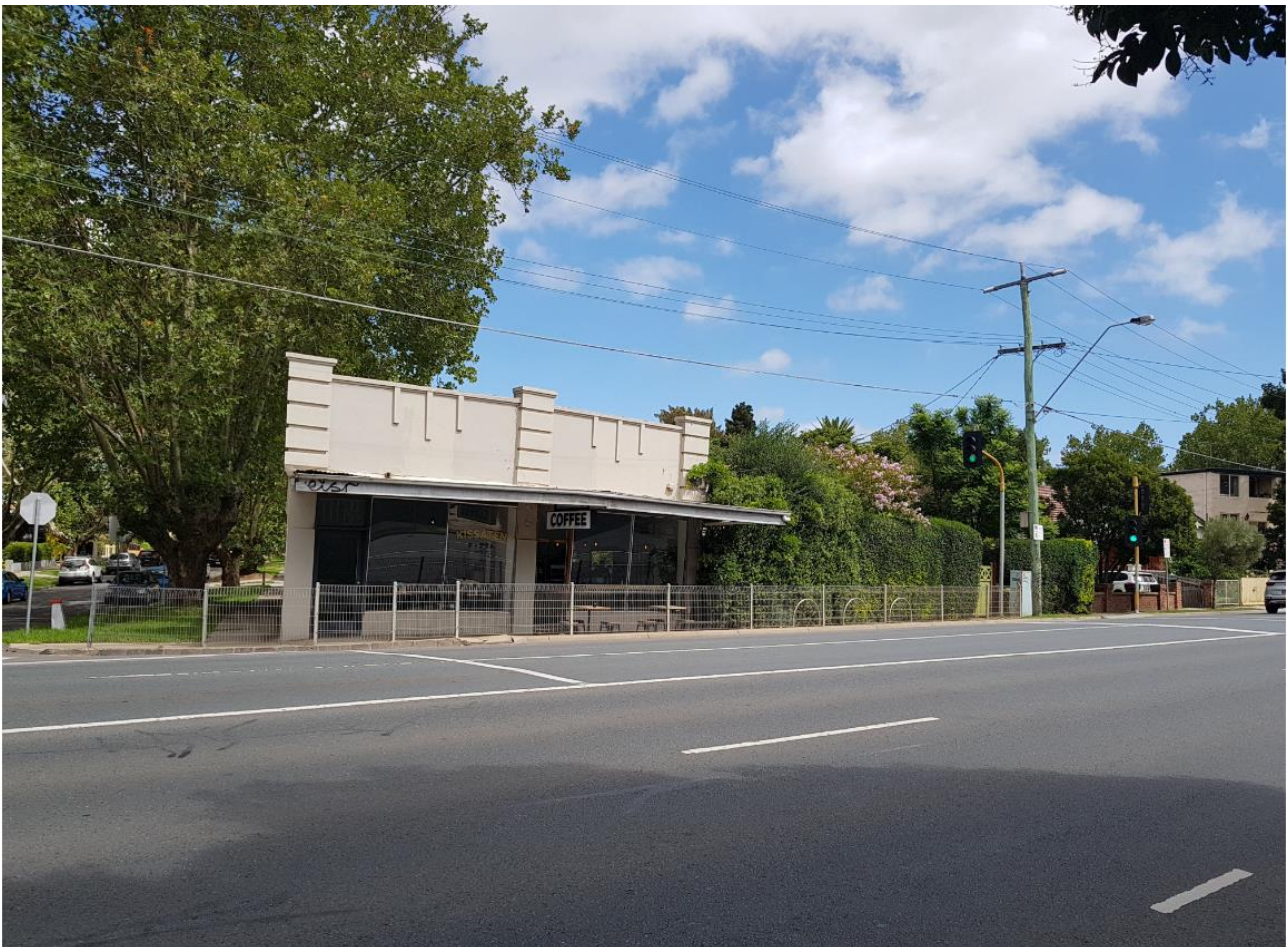
Figure 1 – View of subject site from Heidelberg Road (March 2020)
