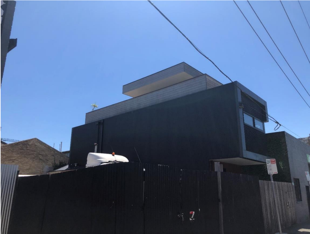
Figure 3: Triple storey dwelling at No. 29 Russell Street (photo taken by Officer on 8/11/2020).
