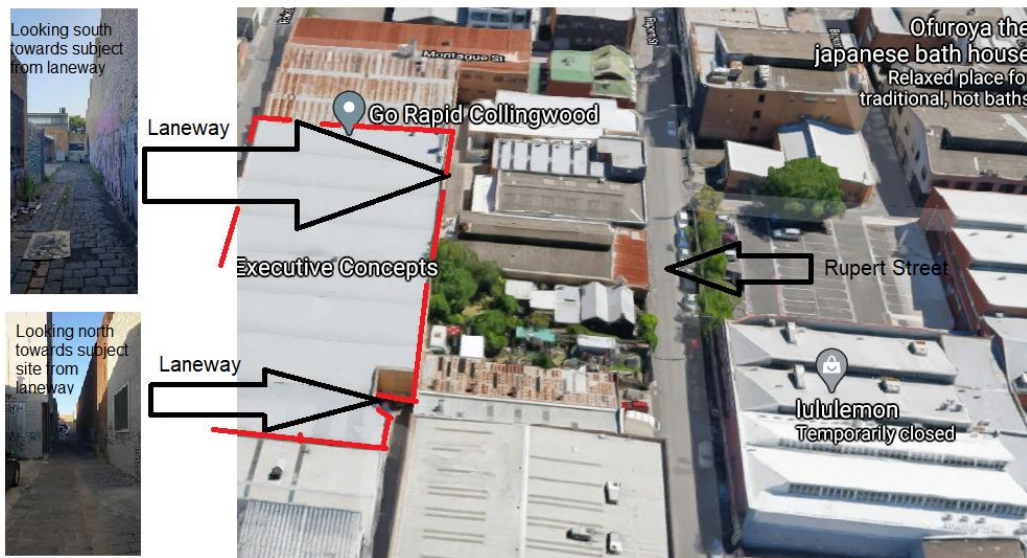
Figure 20: Aerial identifying western context of Rupert Street to the east of the Subject site and two laneways.
