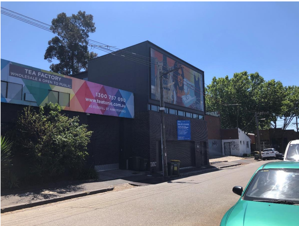
Figure 4: Triple storey office at No. 47 Russell Street (photo taken by Officer on 8/11/2020).
