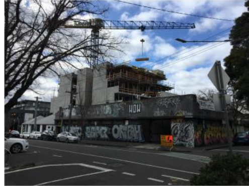
04 Subject Site - Cnr Napier & Chapel St
