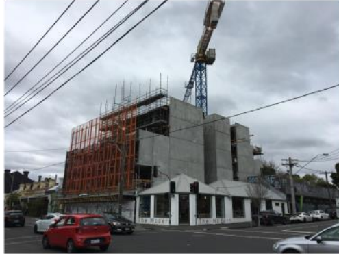
01 Subject Site - Cnr Napier & Johnson St
