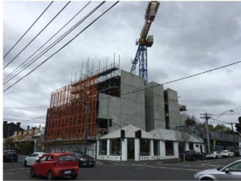
01 Subject Site - Cnr Napier & Johnson St
