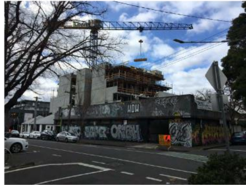
04 Subject Site - Cnr Napier & Chapel St
