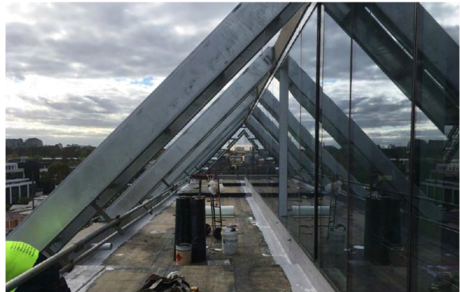
8_VIEW ALONG TERRACE DURING CONSTRUCTION - MAY 2020.
