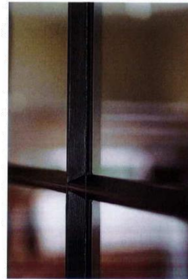
STEEL FRAME WINDOWS FOR HERITAGE WALL 25% TRANSPARENCY ETCHED GLASS TO LOWER PANEL 1g) HERITAGE FACADE FENESTRATION
