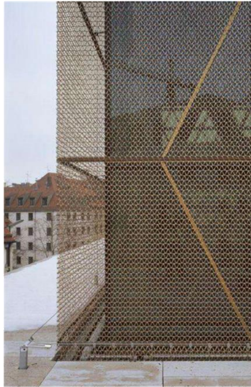
METAL MESH FRAMED ONTO GLAZING.
