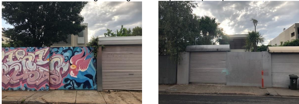
Figure 16: No. 292 Lennox Street and No. 298 Lennox Street (Source: Officer image, taken 18/02/2020)
