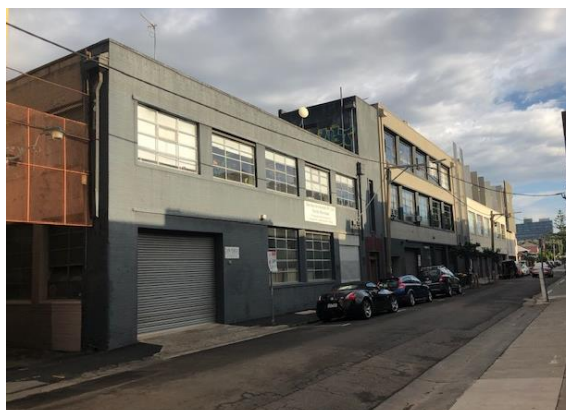
Figure 17: The western side of Wangaratta Street (Source: Officer image, taken 18/02/2020)
