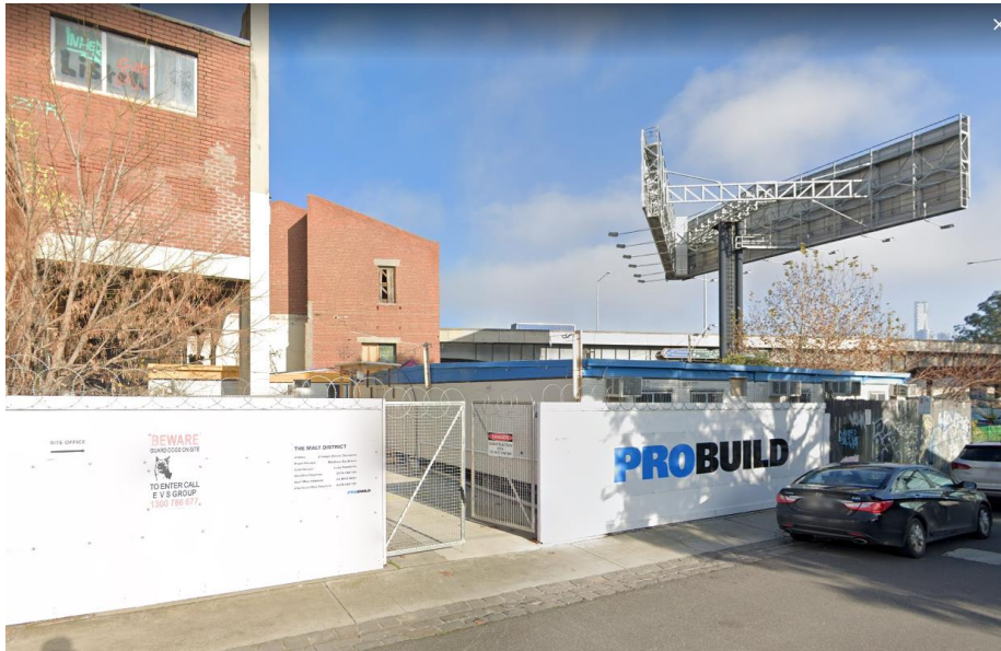
Figure 32 – Gough Street crossover
