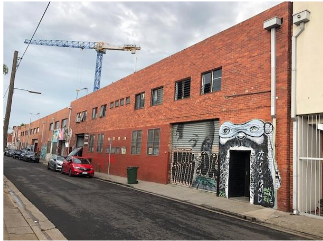
Figure 5: Northern building existing conditions (Botherambo Street) (Source: Officer image, taken 18/02/2020)
