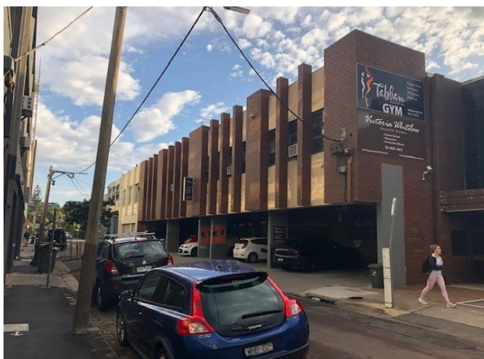
Figure 4: Northern building existing conditions (Wangaratta Street) (Source: Officer image, taken 18/02/2020)
