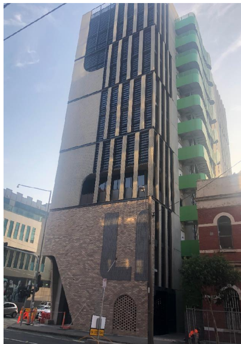
Figure 17: 51 Langridge Street (Wellington Street elevation)
