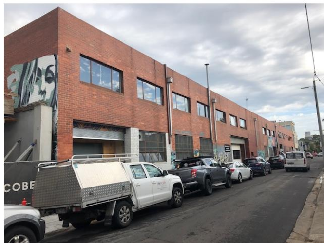
Figure 7: Southern building existing conditions (Botherambo Street) (Source: Officer image, taken 18/02/2020)
