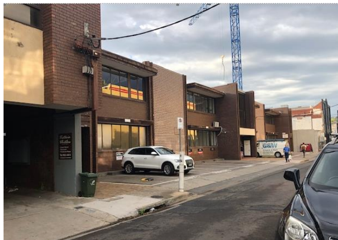
Figure 6: Southern building existing conditions (Wangaratta Street) (Source: Officer image, taken 18/02/2020)
