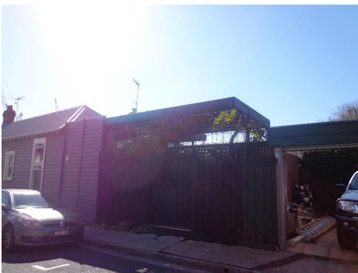
Figure 8 – Rear setback of No. 165 Cubitt Street (with pergola structure visible)
