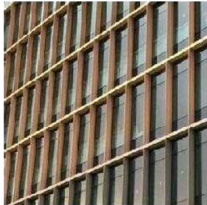
EM-01 ALUMINIUM EXTERNAL SHADING POWDERCOATED TERRACOTTA
