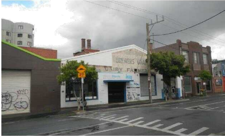
Figure 3 A similar view of the Victoria Old Distillery further south. Note that the white gabled building has painted signage "Brewers Grain". This building should be researched and included in the interpretation signage.
