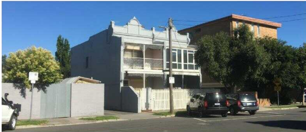
Above: View from Adam Street, within the heritage overlay area
