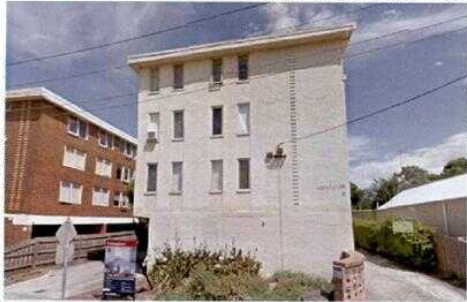
#4. 6 ADAM STREET THREE STOREY BRICK BUILDING
