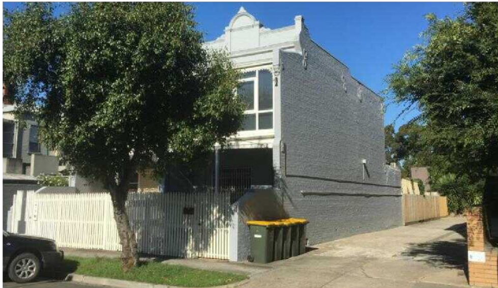
Above: View from Adam Street from outside the heritage area , along the driveway of adjacent property (no. 7 Adam Street)
