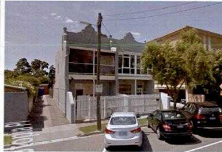
#2. 1-3 ADAM STREET DOUBLE STOREY BRICK TERRACE HOUSES
