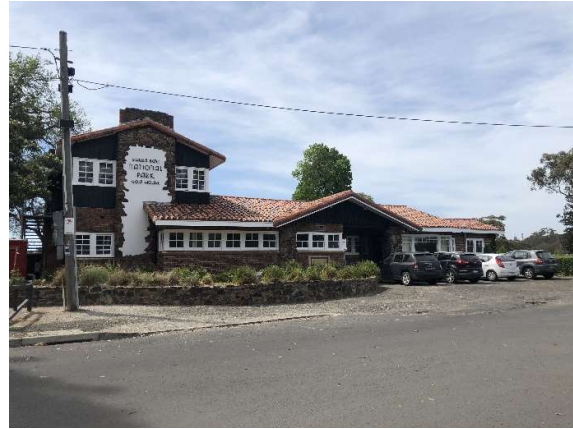
2019, SE facing image showing the 1936 golf club house.
