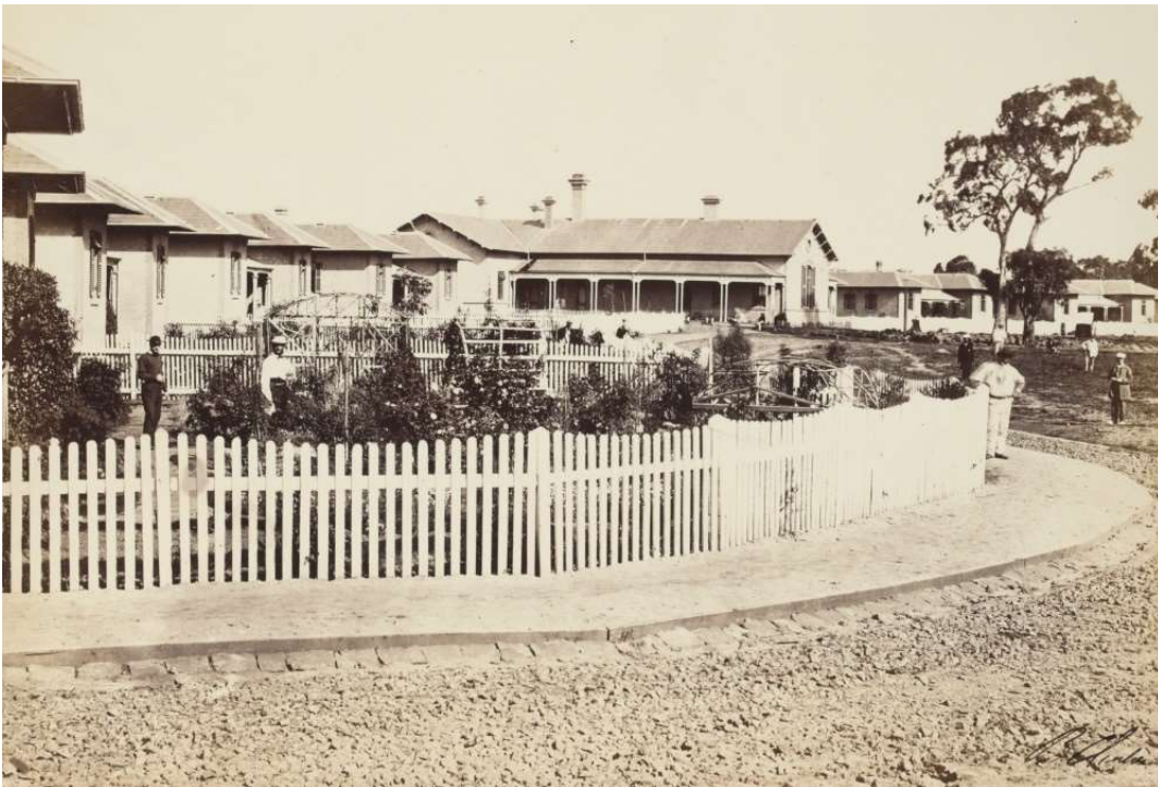
1861, Photograph showing cottages at Yarra Bend Asylum. Source SLV
