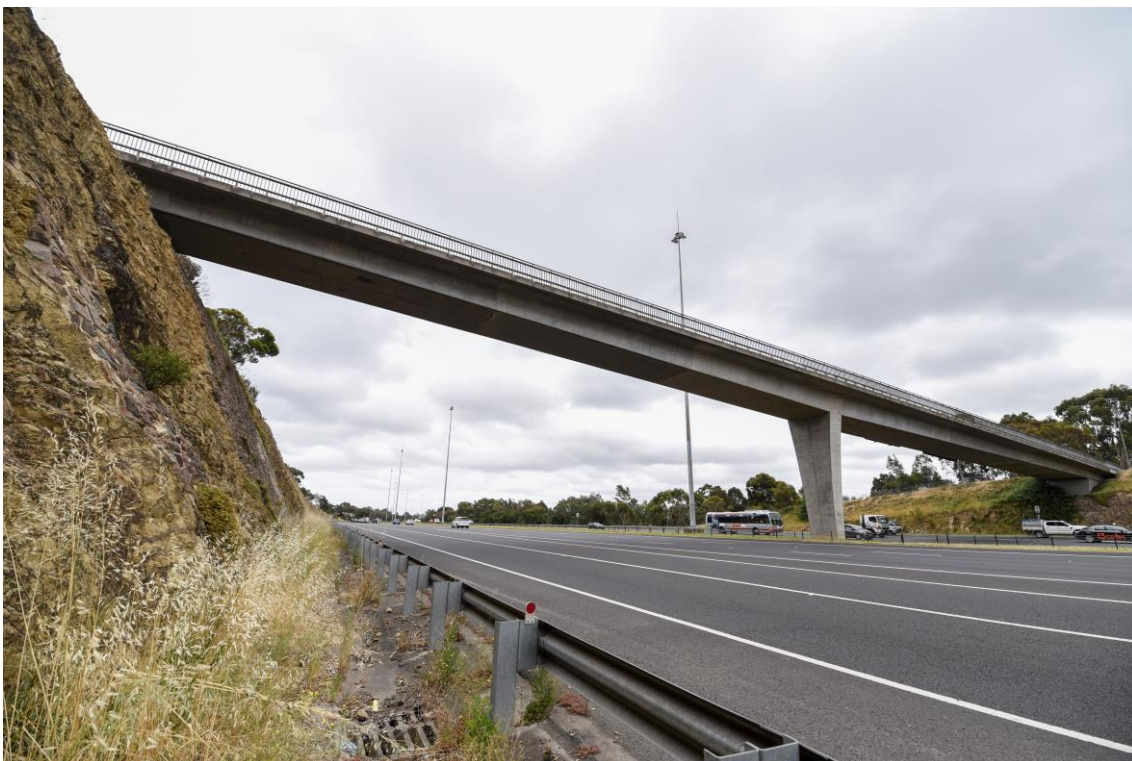
2019, Columba Street overpass, North Balwyn.
