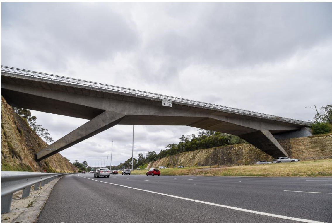
2019, Belford Road overpass at Kew East.
