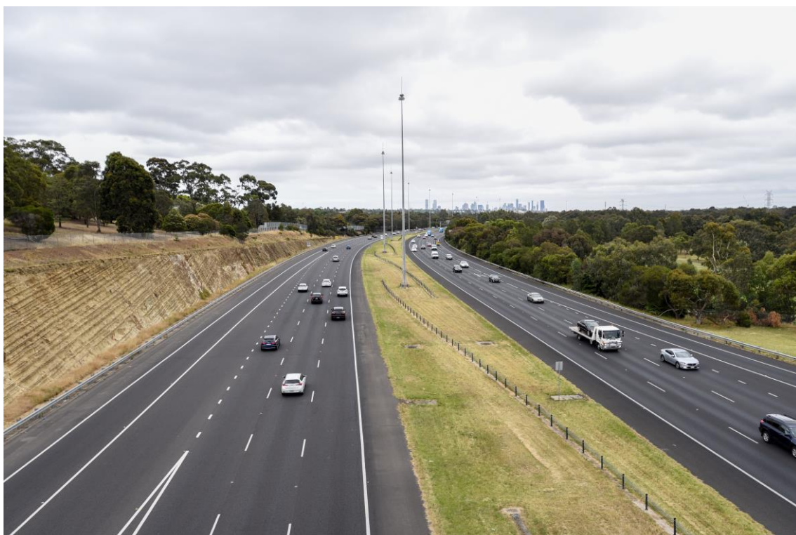
2019, View from Columba Street overpass, looking west.
