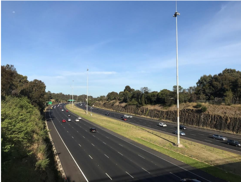
2019, Looking east from Yarra Bend Road Bridge.
