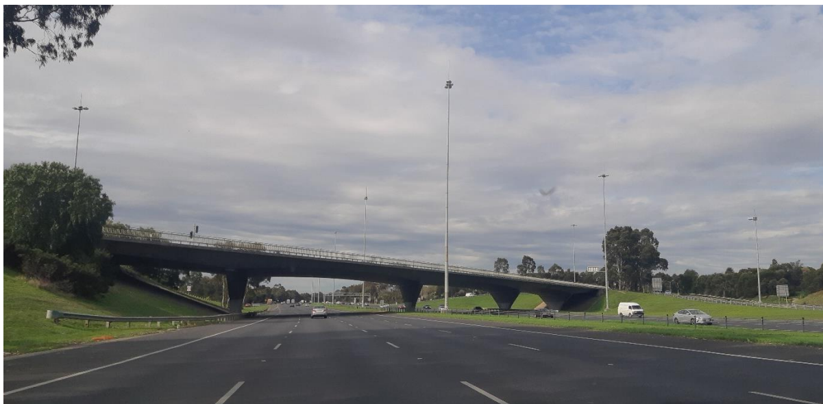
2019, Chandler Highway overpass.
