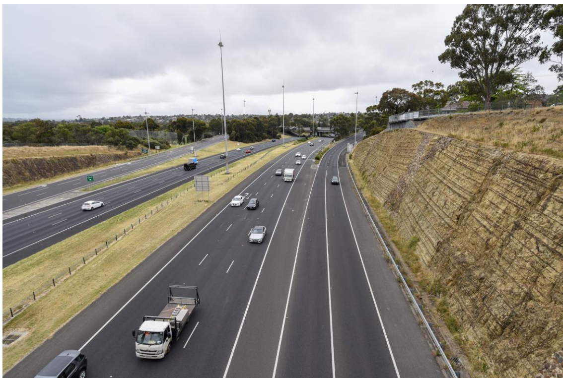
2019, Bulleen Road exit, looking east.
