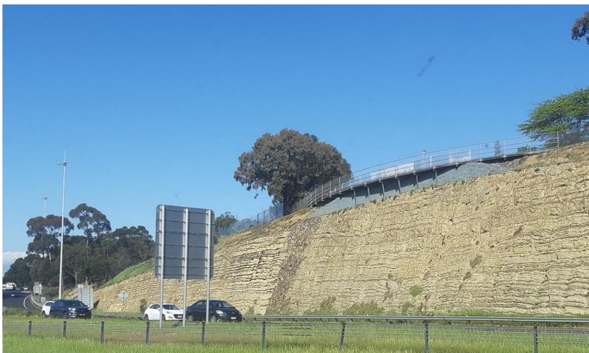
2019, Exposed escarpment and mortared rock infill, just east of the Columba Street overpass, North Balwyn.
