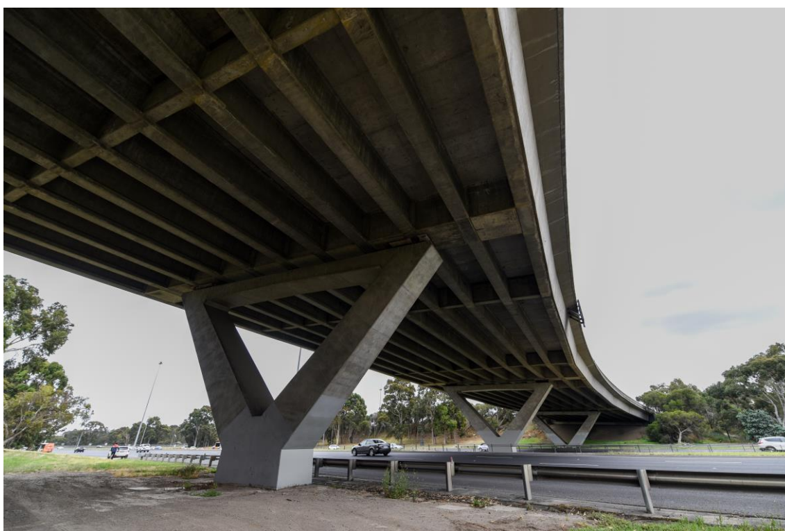
2019, Burke Road overpass, Looking northwest.
