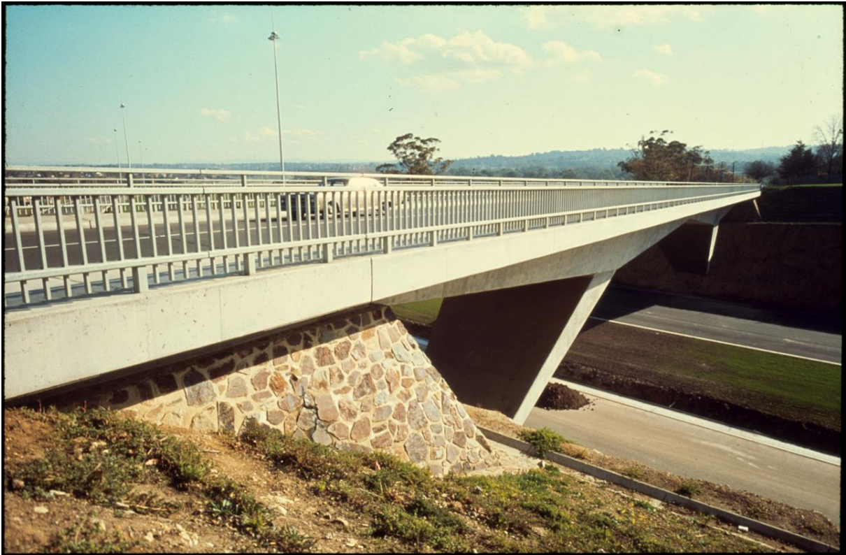
1976, Belford Road Bridge, prior to the opening of the Eastern Freeway - Stage One. Source: National Archives of Australia.
