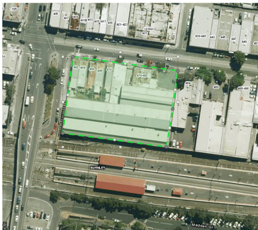
Map 1: aerial photo showing subject land, 462-482 Swan Street, Richmond
