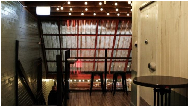
Fig.4 The first floor deck above the courtyard (facing south).
