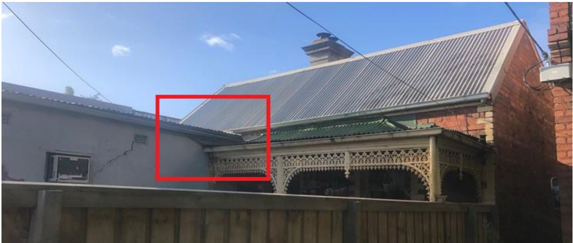
Figure 10: The front-verandah of the Victorian-era dwelling has been altered to make way for the Inter-war-era shop building.
