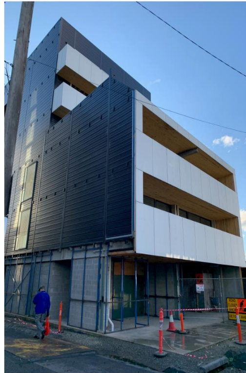
Figure 2: Huckerby Street view of subject site.
