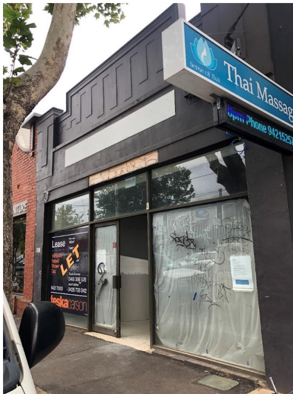
Image 1: The subject site as it appears to Swan Street.
