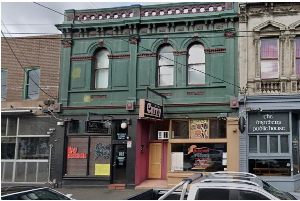
Fig.1 The Johnston Street frontage of the site.
