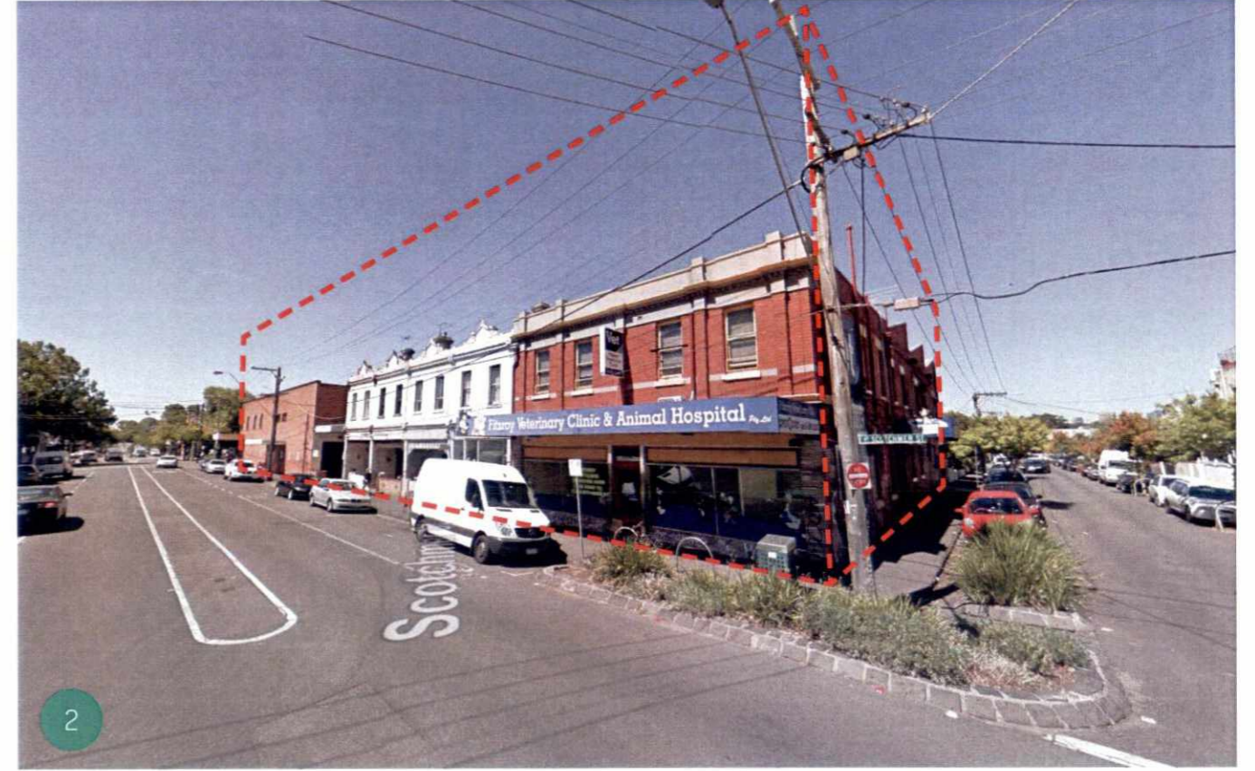
Photograph 02 - View from corner of Scotchmer St and Egremont St
