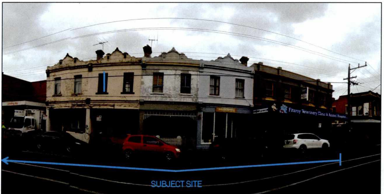
Figure 2.7 VIEW OF SUBJECT SITE – SCOTCHMER STREET FRONTAGE
