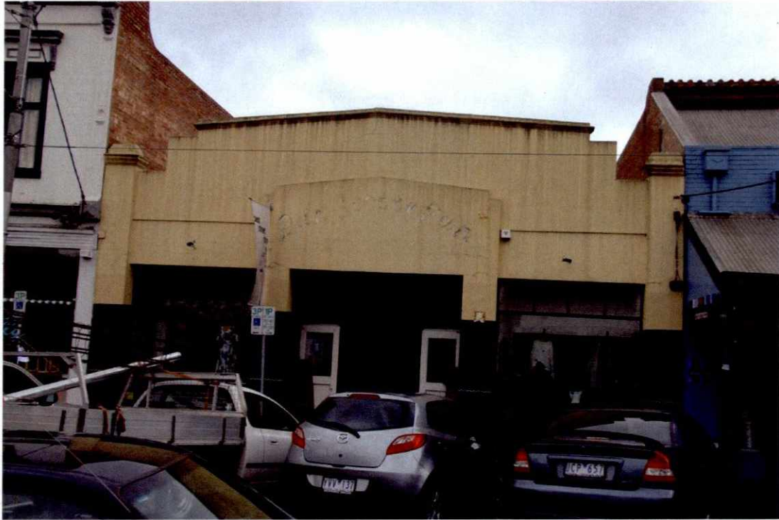
Figure 16 Former J Fisher and Co motor workshop at 31-33 Best Street
