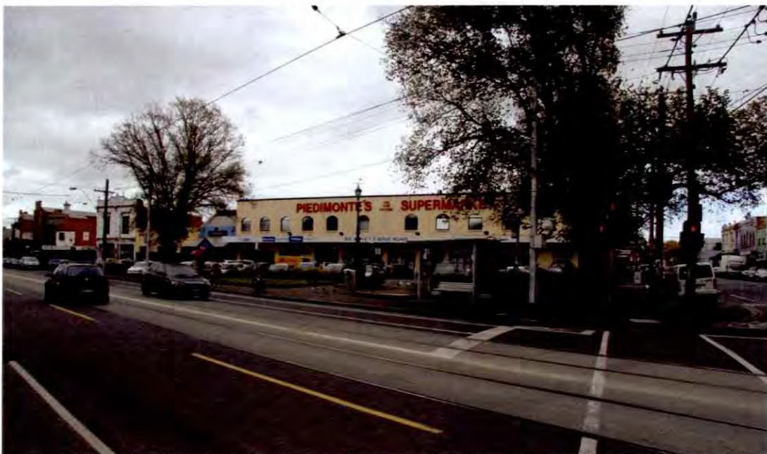
Figure 13 View from St. Georges Road of subject properties on Best Street
