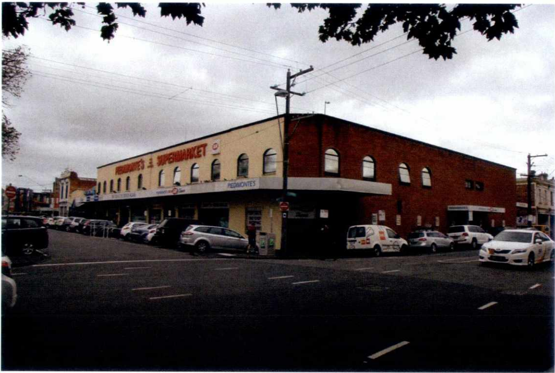
Figure 18 View of Piedimonte's Supermarket from the corner of Best and Scotchmer streets
