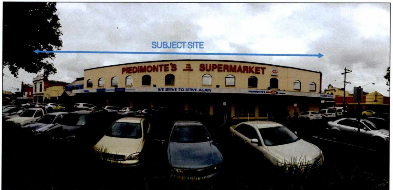
Figure 2.5 VIEW OF SUBJECT SITE – BEST STREET FRONTAGE
