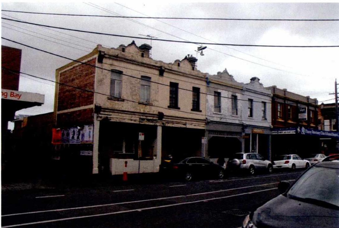
Figure 8 108-114 Scotchmer Street with the side (east) wall to laneway evident
