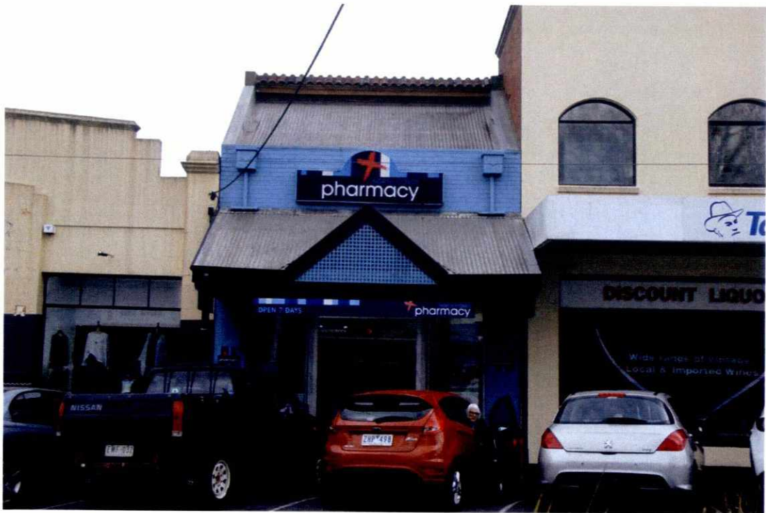
Figure 15 Former residence, now commercial building at 35 Best Street
