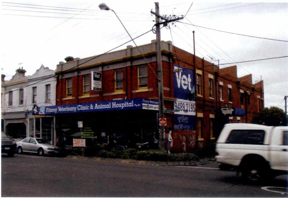
Figure 7 102-106 Scotchmer Street with side elevation to Egremont Street evident
