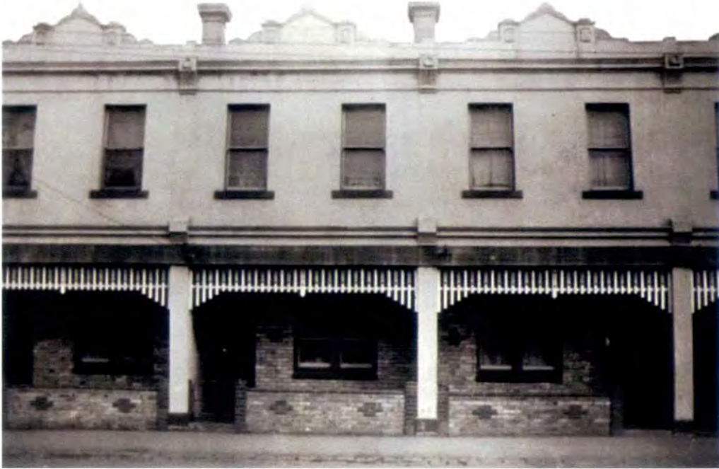
Figure 5 1948 photograph of the terraces along Scotchmer Street, showing changes to the ground floor facades following their conversion to residential use Source: Yarra Libraries
