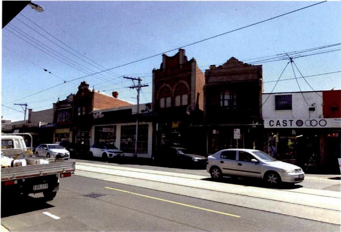
Figure 20 View of St. Georges Road to the south of the subject site
