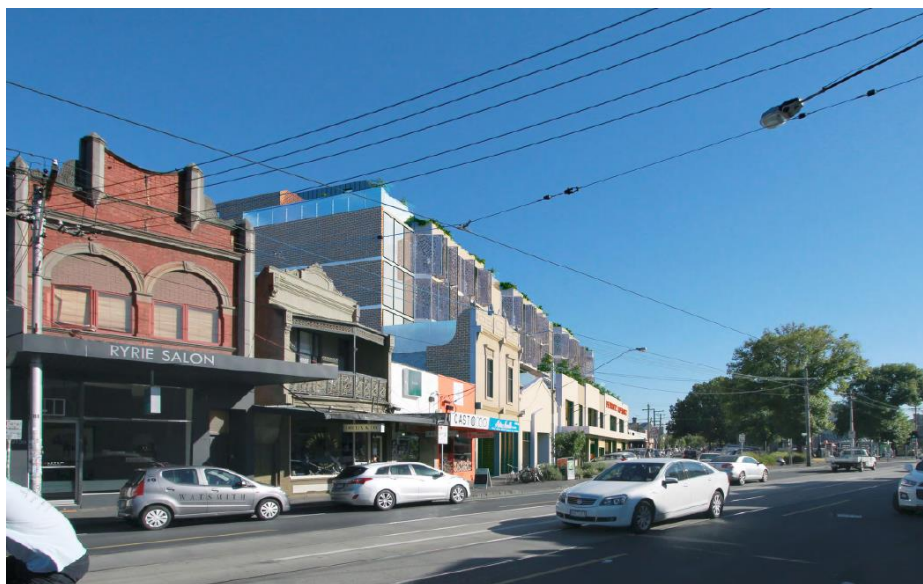
Figure 5: Looking from the south, from along St Georges Road, towards the southern side of the proposal
